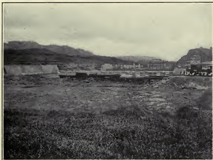
FIG. 17.—SPILLWAY CHANNEL DURING CONSTRUCTION, GATUN, CANAL ZONE.
