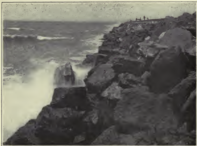
FIG. 6.—TORO POINT BREAKWATER, LOOKING TOWARDS WATER END, JULY 12. 1913.
