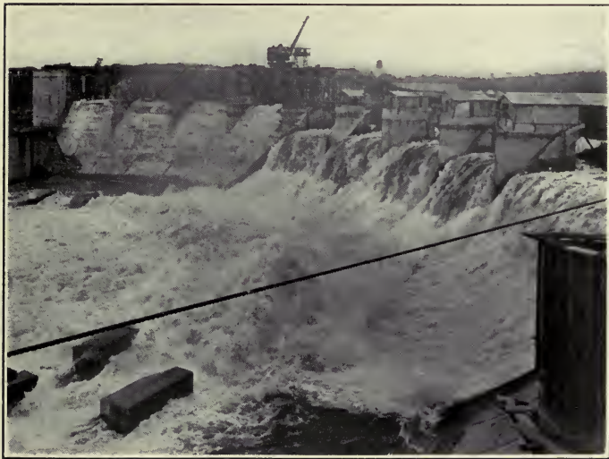
FIG. 19.—FLOOD WATER PASSING OVER INCOMPLETED SPILLWAY DAM AT GATUN.
