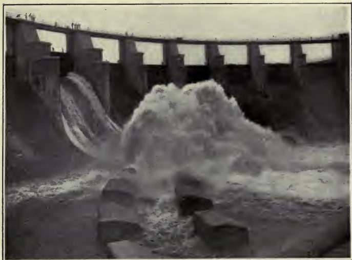
FIG. 4.—THE OPENING OF THE FIRST GATE, GATUN SPILLWAY.
