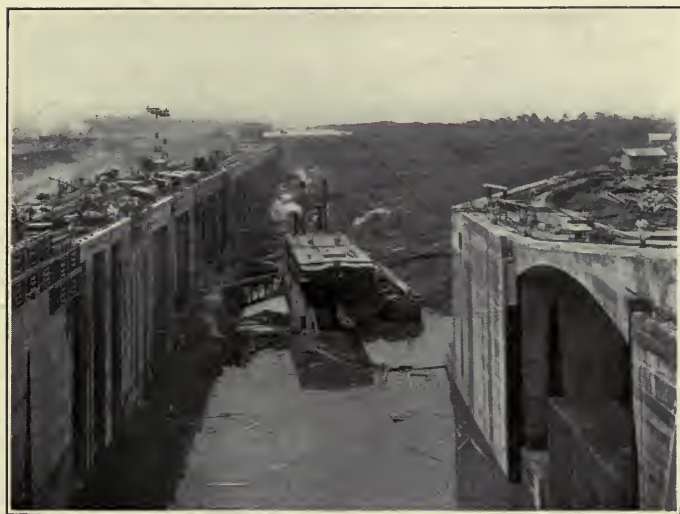
FIG. 7.—A DREDGE GROUNDED FIFTY-FIVE FEET BELOW SEA-LEVEL, GATUN LOCKS.
