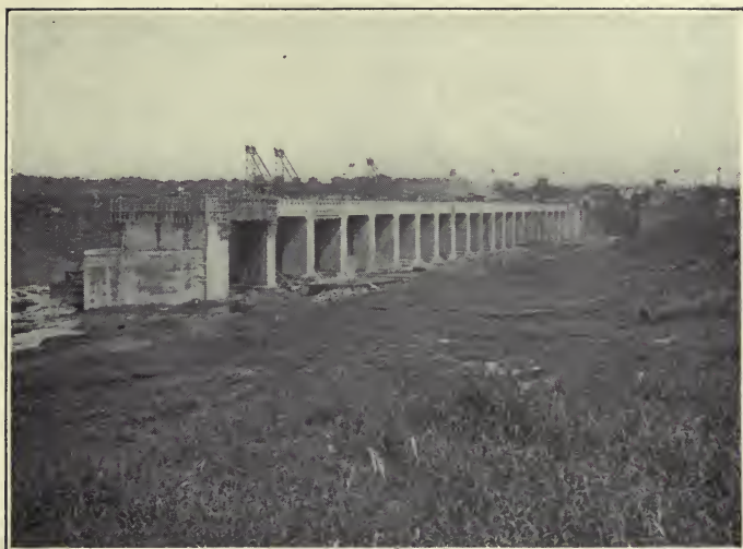
FIG. 1.—NORTH GUIDE WALL, GATUN LOCKS.
