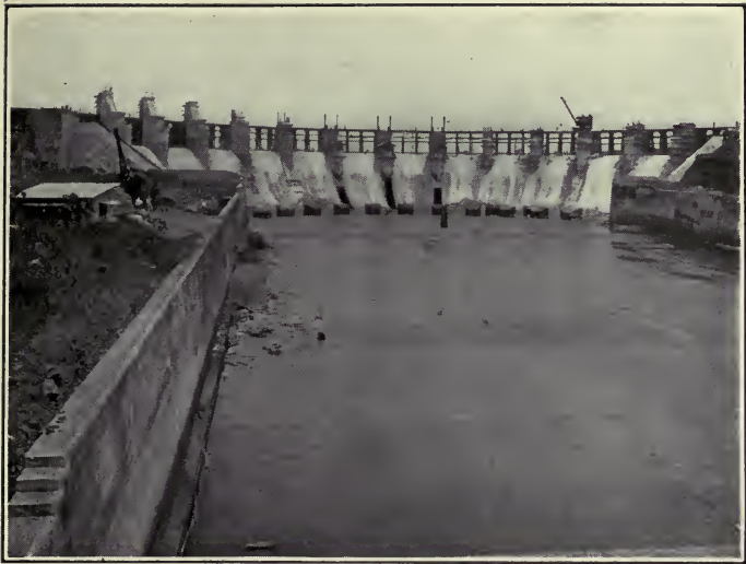
FIG. 18.—GATUN SPILLWAY DAM UNDER CONSTRUCTION.
