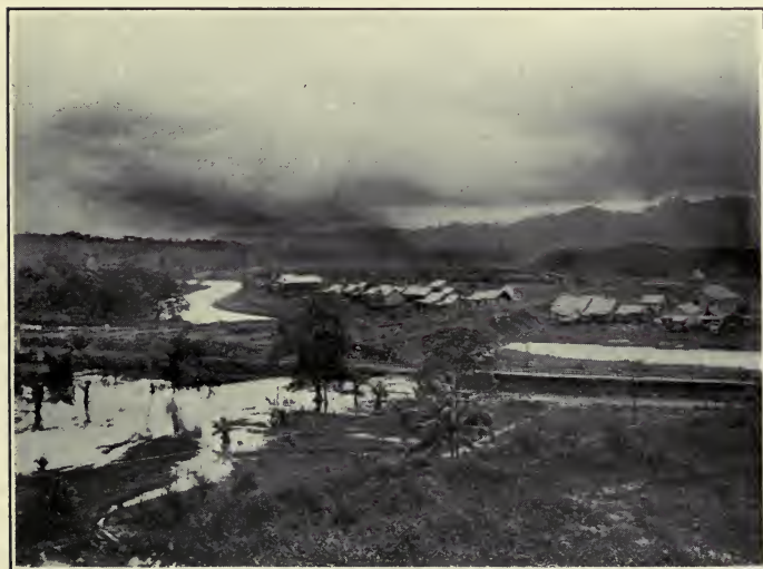
FIG. 2.—DAM CONSTRUCTION THROUGH GATUN VILLAGE.
