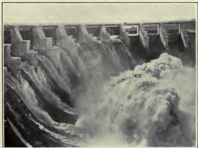
FIG. 5.—GATUN SPILLWAY WITH SEVEN GATES OPEN.
