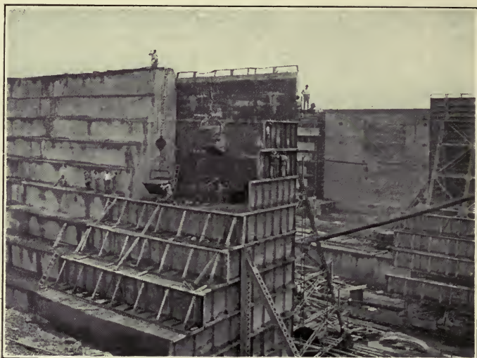
CLOSE VIEW OF STEEL FORMS, GATUN LOCKS.
