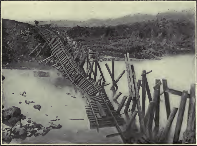
FIG. 12.—REMAINS OF THE NORTH DIVERSION DAM, GATUN DAM.
