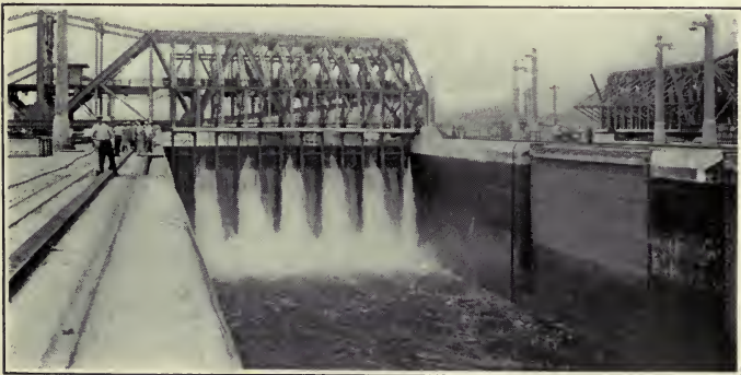
FIG. 3.—VIEWS OF EMERGENCY DAM AT GATUN IN OPERATION.
