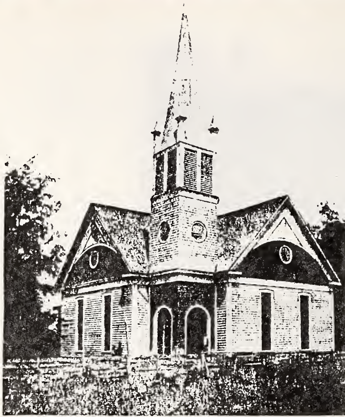
EAST BEND METHODIST CHURCH
