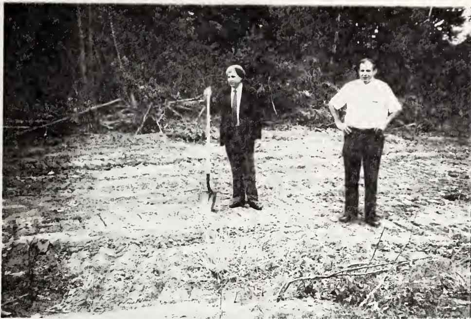
OUR HOPES AND DREAMS FOR FUTURE GROWTH..... GROUND BREAKING AUGUST 25TH, 1987 EAST BEND INDUSTRIAL PARK
