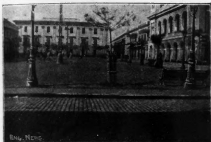
Plaza at San Juan, Porto Rico, Showing Slag-brick Paving in Foreground, with Plaza Covered with Concrete.
