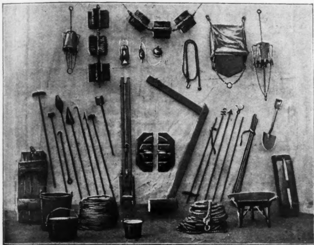
FIG. 3.—TOOLS FOR REMOVING OBSTRUCTIONS.
