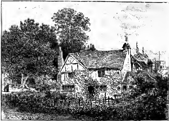
MILTON'S COTTAGE, FROM THE FIELD AND HILLSIDE ADJOINING IT, CHALFONT-ST.-GILES.
