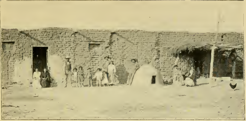
FIG. 1.—A ROW OF ADOBE HOUSES IN NEW MEXICO.
