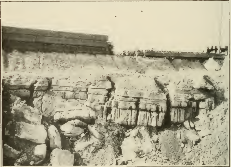
Fig. 6. Joints enlarged by solution. Cut on Illinois Central R. R., Bloomington.
