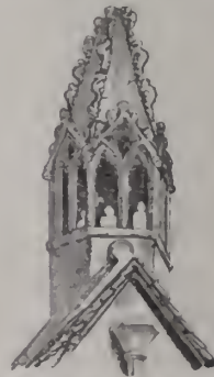
Chimney, Barford, Oxfordshire.
