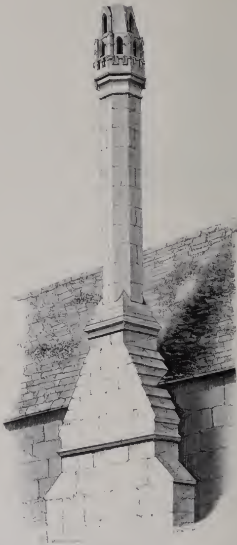
CHIMNEY. ARCHBISHOP'S PALACE, SOUTHWELL, NOTTINGHAMSHIRE
