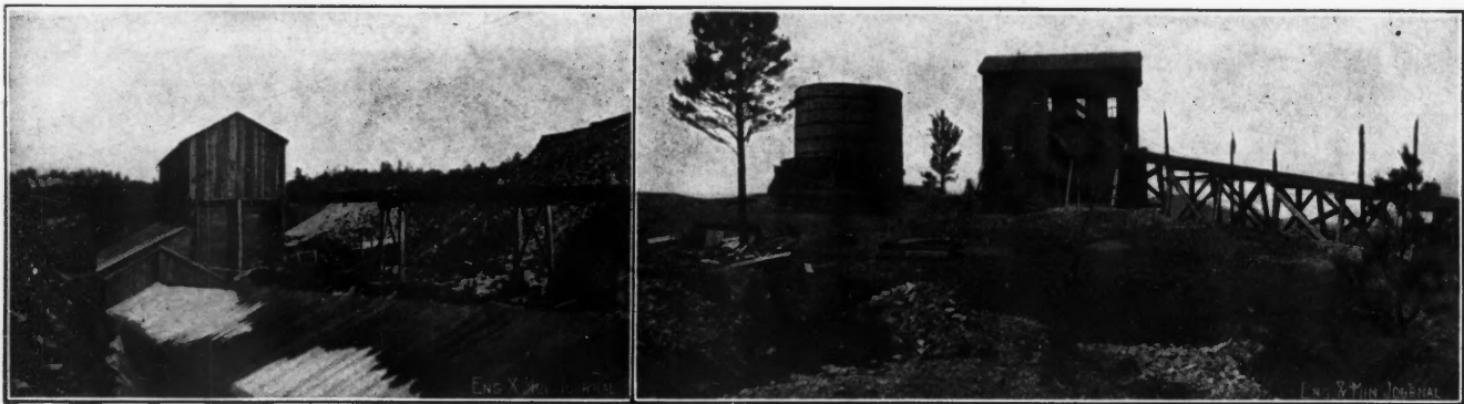
ORE FROM THE SOUTH SIDE IS DUMPED INTO THE ORE BIN ON THE LEFT DURING THE DAY AND AT NIGHT IS HOISTED IN SKIPS AND AUTOMATICALLY DUMPED INTO THE MILL BINS SHOWN AT THE RIGHT
