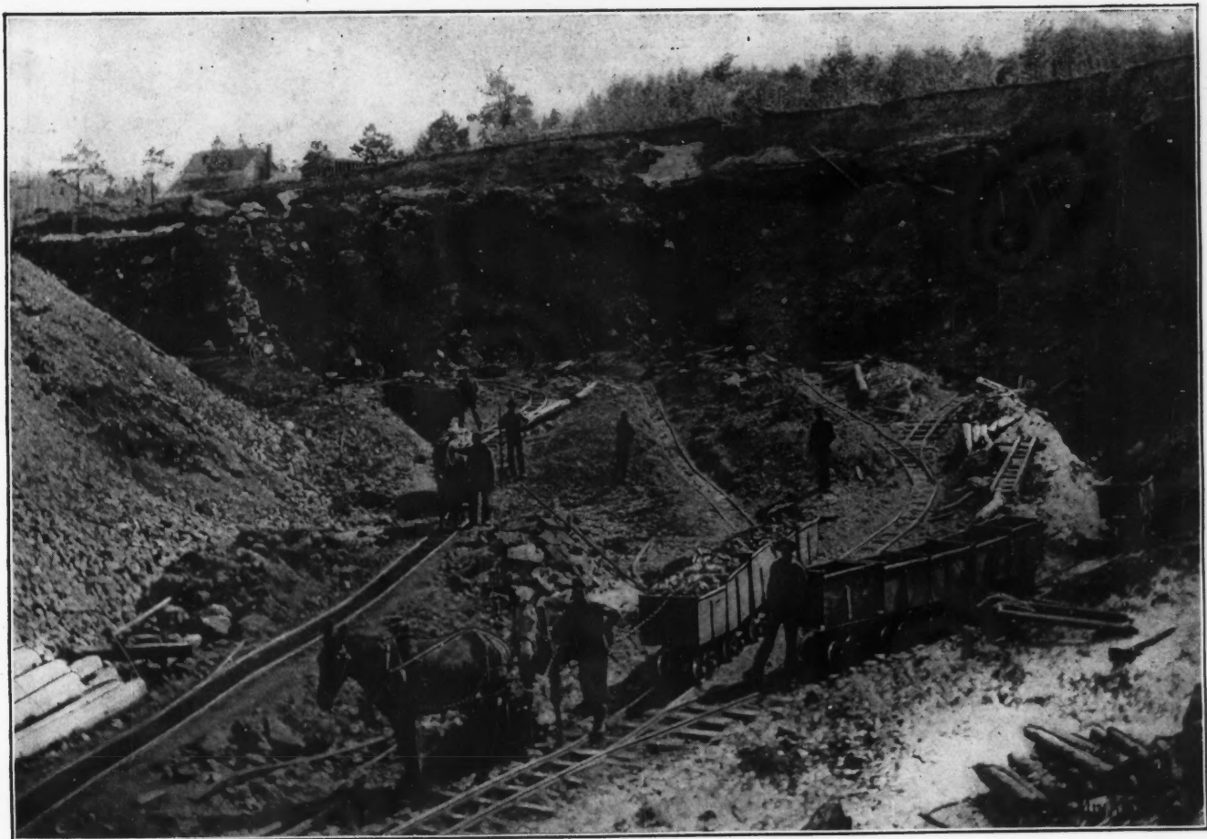
TRAMMING ORE FROM THE SOUTH SIDE OF THE WASP OPENCUT
