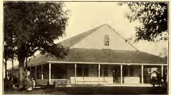
SHELTER HOUSE IN EAGLE POINT PARK
