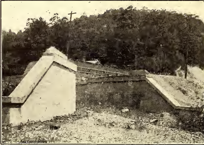
PLATE GIRDER BRIDGE WITH CONCRETE ABUTMENTS
