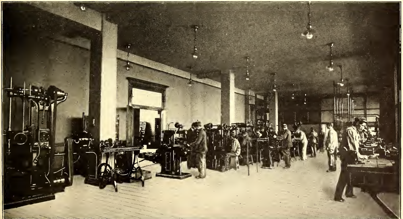
GENERAL VIEW OF MACHINE SHOP ON THIRD FLOOR, SHOWING INDIVIDUAL MOTOR DRIVE
