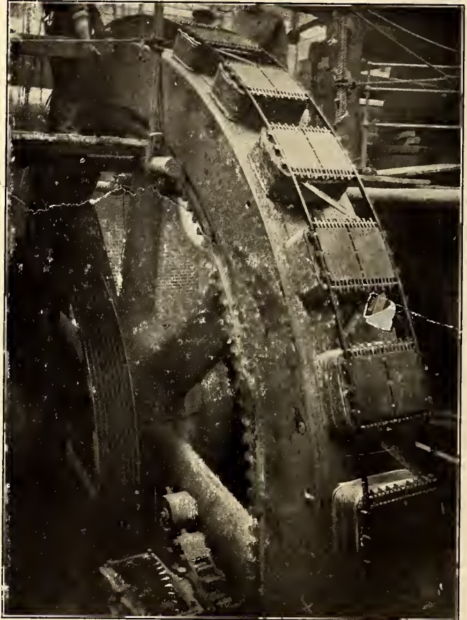
GENERATOR BEING INSTALLED
