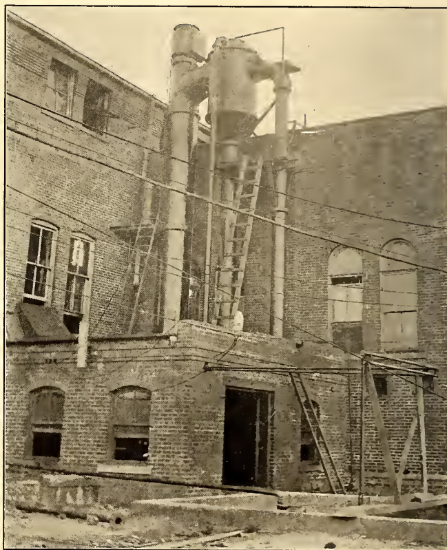
CONDENSER INSTALLATION FOR VERTICAL TURBINE
