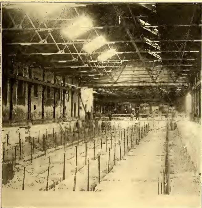
TWISTED RODS IN POSITION FOR CONCRETING TO FORM THE PIT PIERS
