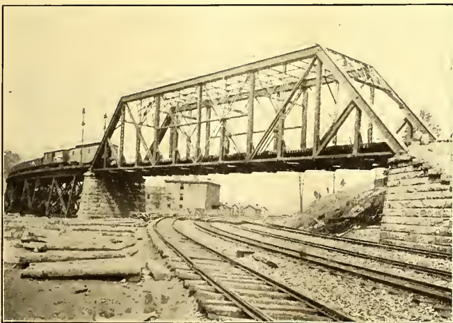
UNION RAILROAD BRIDGE OVER PENNSYLVANIA RAILROAD TRACKS AT BESSEMER, PA.
