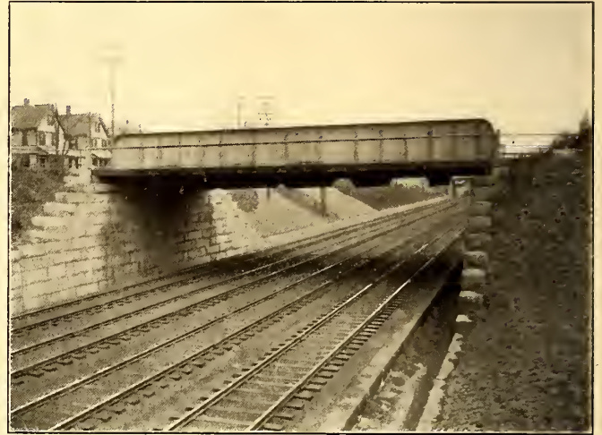
RICHARDSON STREET BRIDGE, NEWTONVILLE, MASS.
