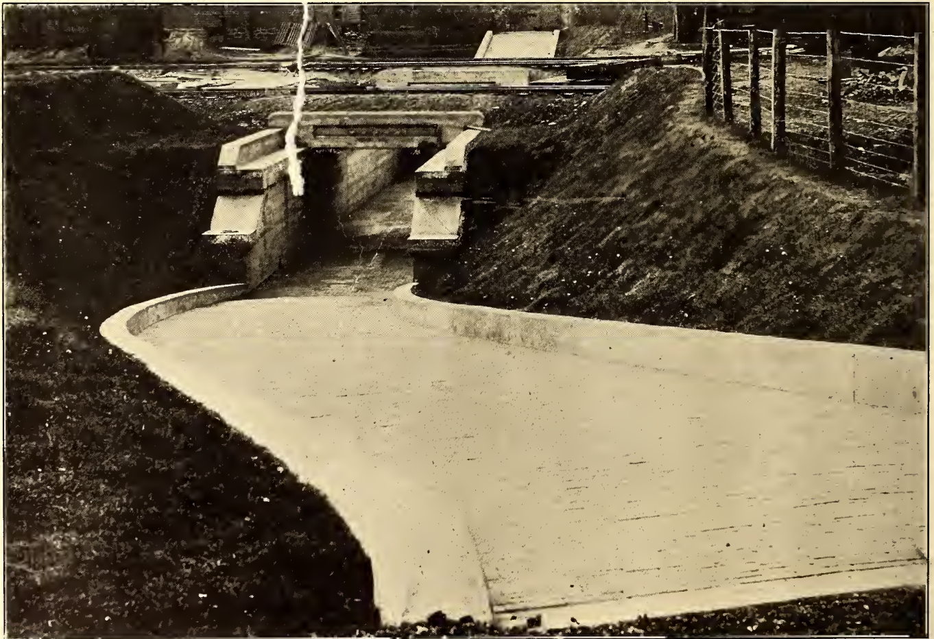
CONCRETE PASSAGEWAY AT GENESSEE VALLEY PARK, ROCHESTER
