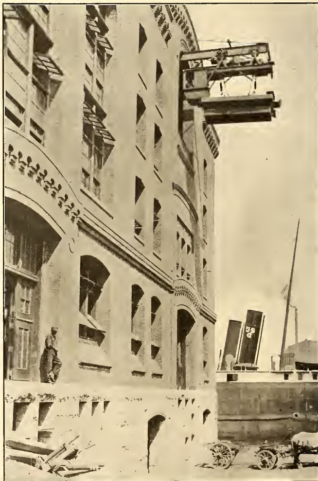
A WAGON BED LOADED WITH COAL BEING ELEVATED BY THE CRANE
