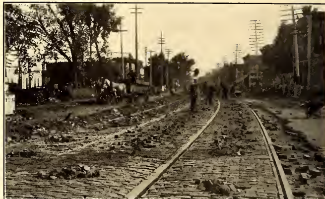
LAYING THE PAVEMENT
