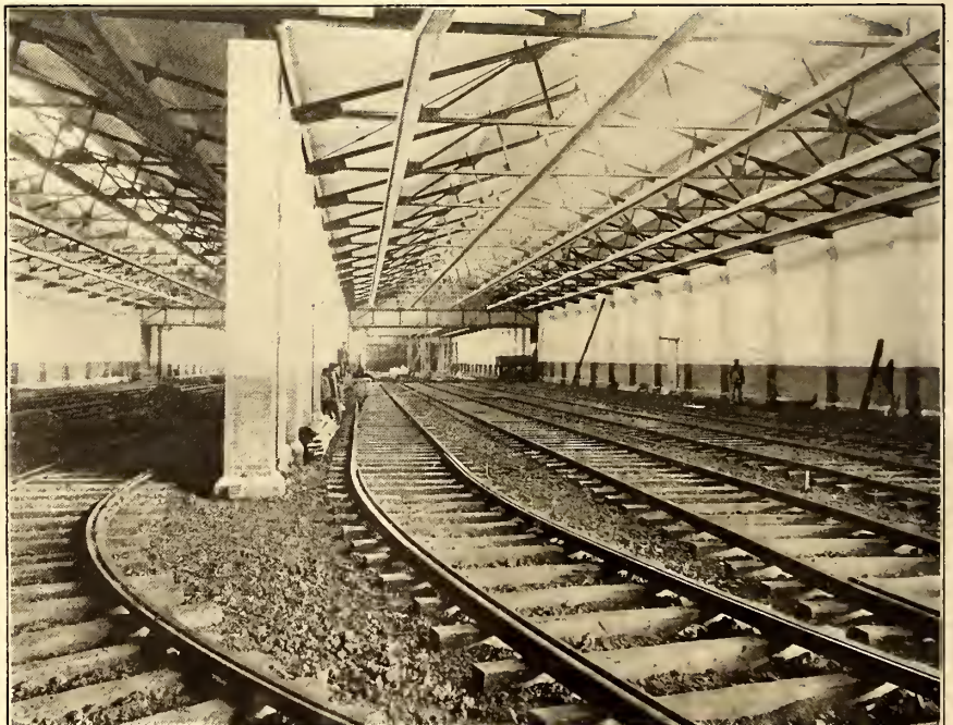
VIEW FROM SAND DRIER, LOOKING TOWARD MASTEN STREET, OR REAR END OF CAR HOUSE
