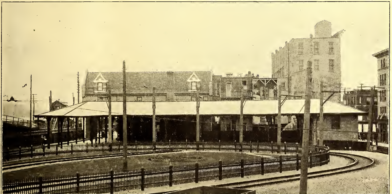
WILKESBARRE TERMINAL STATION, FROM YARD SIDE
