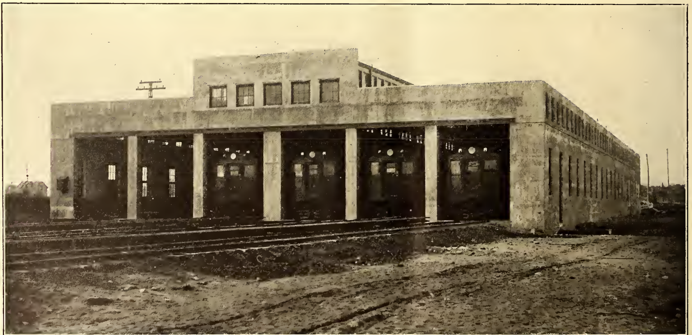
FIG. 28.—EXTERIOR OF DUNTON INSPECTION SHED
