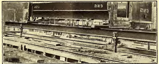
CAR-BODY WEIGHING TWELVE TONS PARTLY RAISED ON JACK LIFT, ARABELLA CAR HOUSE, NEW ORLEANS
