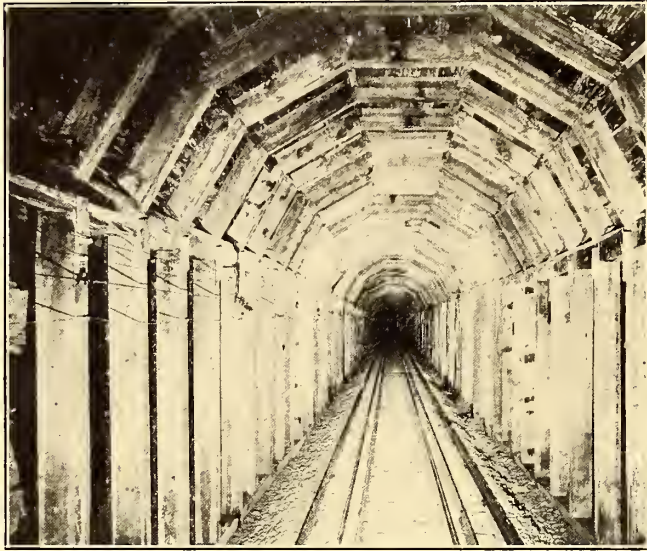
TIMBER SECTION OF TUNNEL
