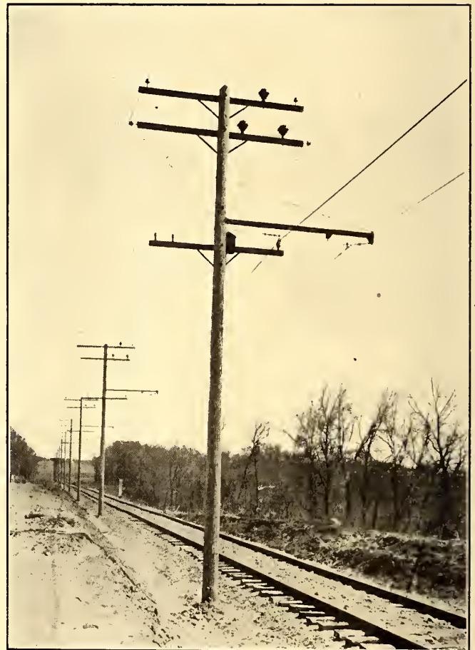
ONE OF THE SPECIAL POLES PLACED EVERY 1000 FT., UPON WHICH LIGHTNING ARRESTERS ARE GROUNDED, TROLLEY FEED-IN TAPS ARE MADE, AND THE HIGH-TENSION GROUND WIRES RUN TO EARTH
