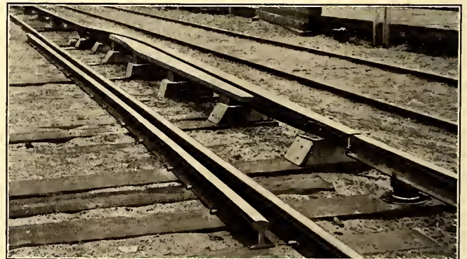
FIG. 16.—CAM IN THIRD RAIL FOR CHANGING ADJUSTABLE SHOE
