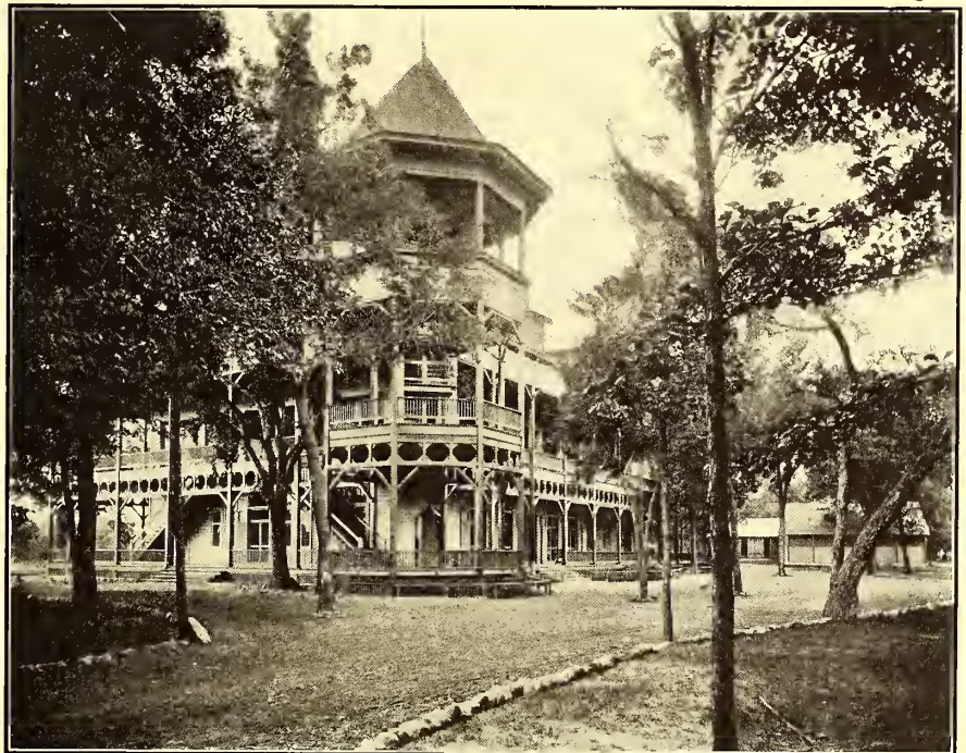
FRONT VIEW OF PAVILION IN RIVERSIDE PARK
