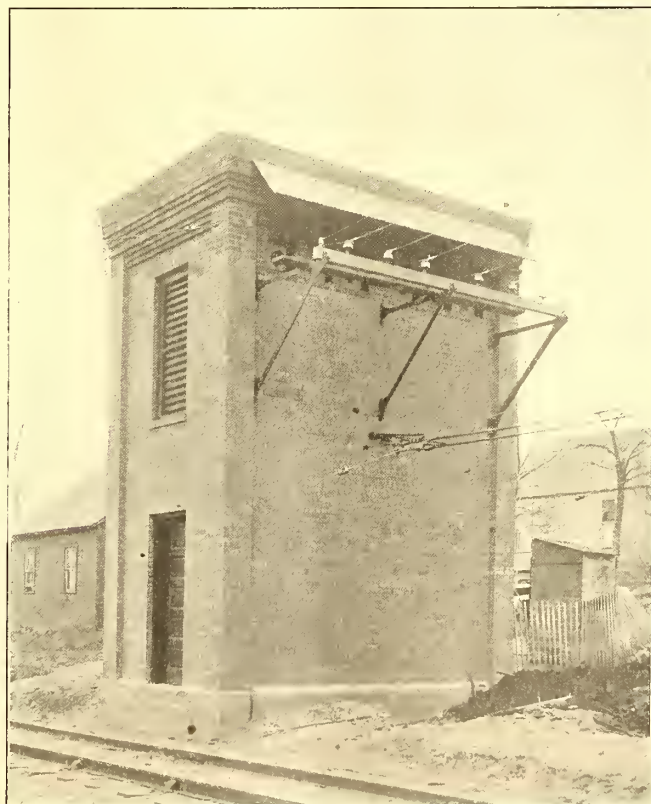
BRICK CABLE HOUSE NEAR CITY LIMITS
