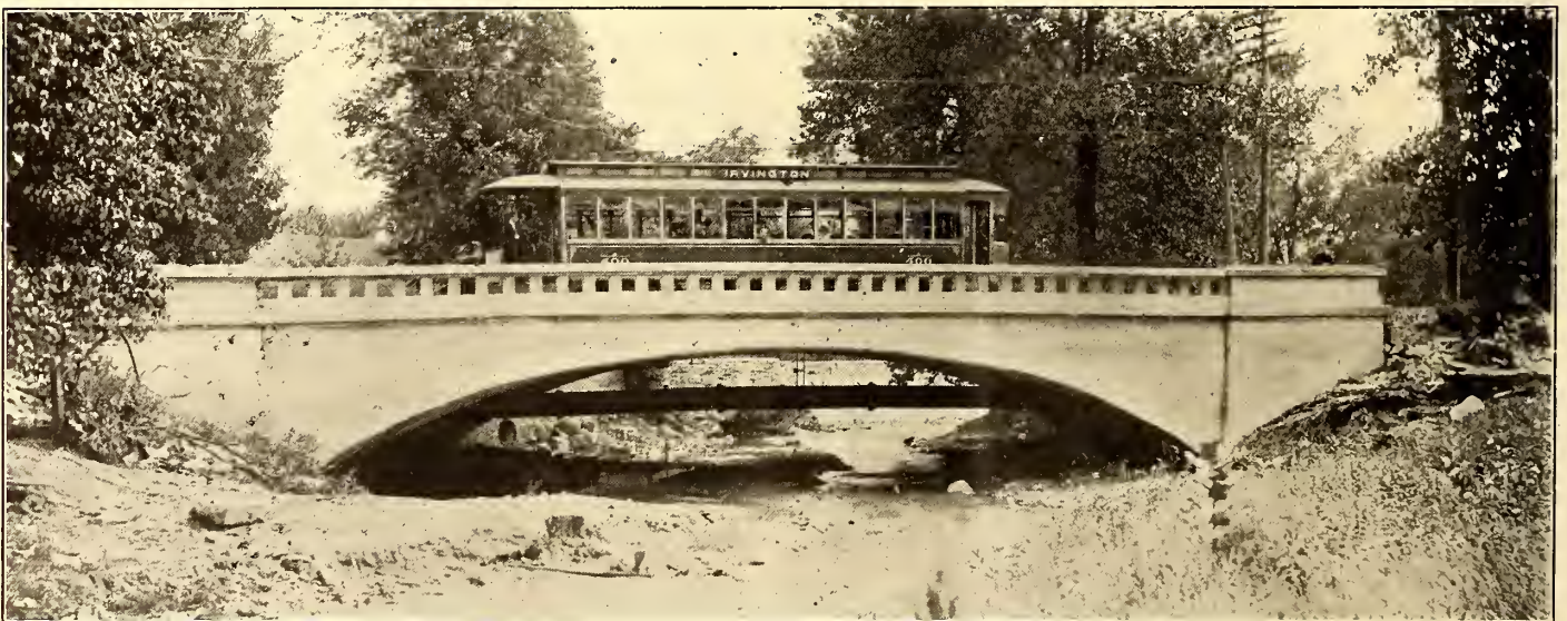
FIG. 8.—A 65-FT. CONCRETE ARCH ON EAST WASHINGTON STREET, INDIANAPOLIS
