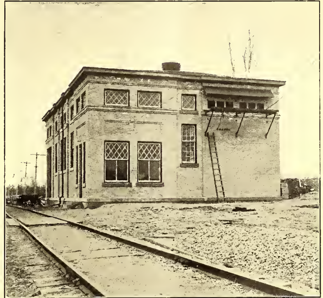
THE EXCELSIOR SUB-STATION
