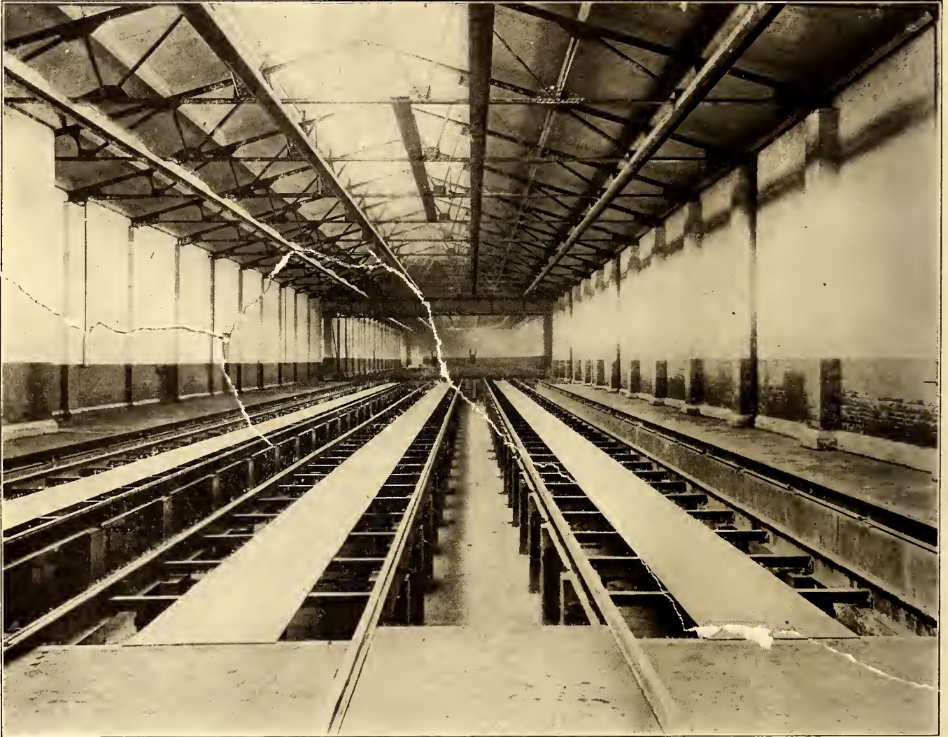
VIEW THROUGH THE CAR HOUSE, SHOWING THE PITS, CHECKER PLATES, RADIATORS AND SKYLIGHT CONSTRUCTION
