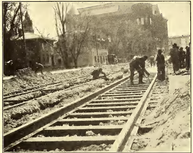
NEW TRACK CONSTRUCTION ON HENNEPIN AVENUE, MINNEAPOLIS
