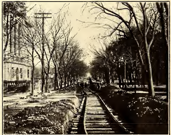
TRACK CONSTRUCTION IN RESIDENTIAL STREET AND OPPOSITE THE STATE UNIVERSITY
