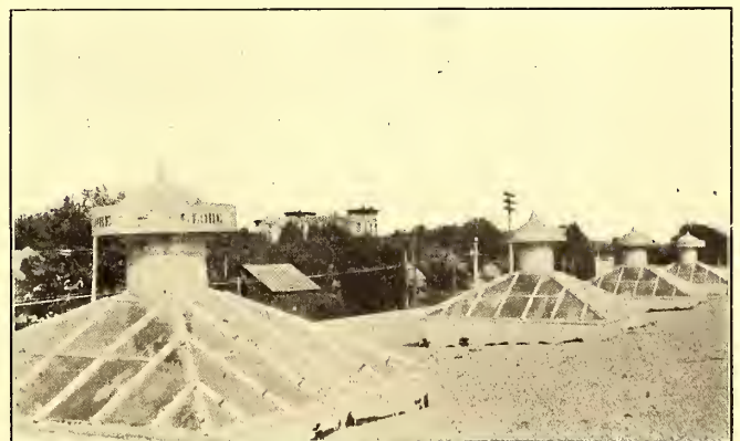
ROOF OF REPAIR SHOP, SHOWING VENTILATORS AND SKYLIGHTS
