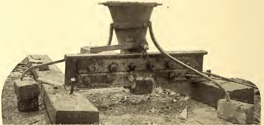
MOLD USED IN WELDING
