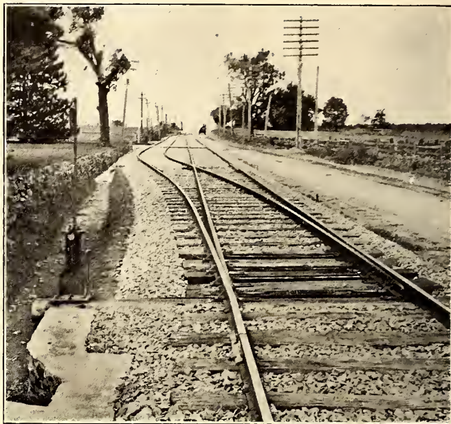
TYPICAL CONSTRUCTION AT A TURNOUT
