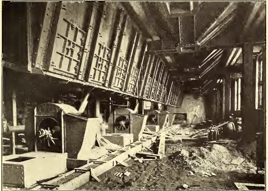
CONSTRUCTION VIEW OF PASSAGE-WAY UNDER THE BOILERS
