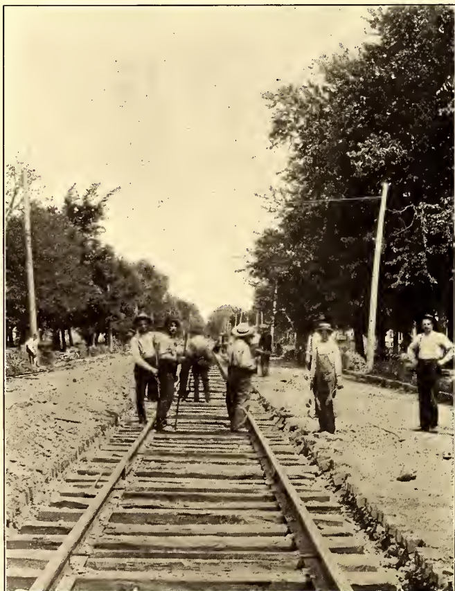
TAMPING UNDER THE TIES
