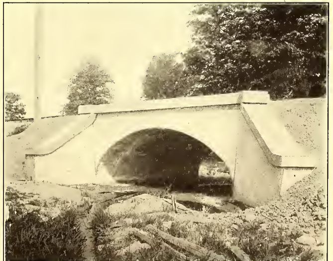
FIG. 4.—A 20-FT. SPAN ON THE INDIANAPOLIS & NORTHERN LINE
