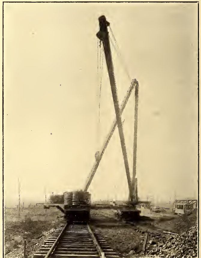
HOME-MADE TRAVELING DERRICK IN CLEVELAND
