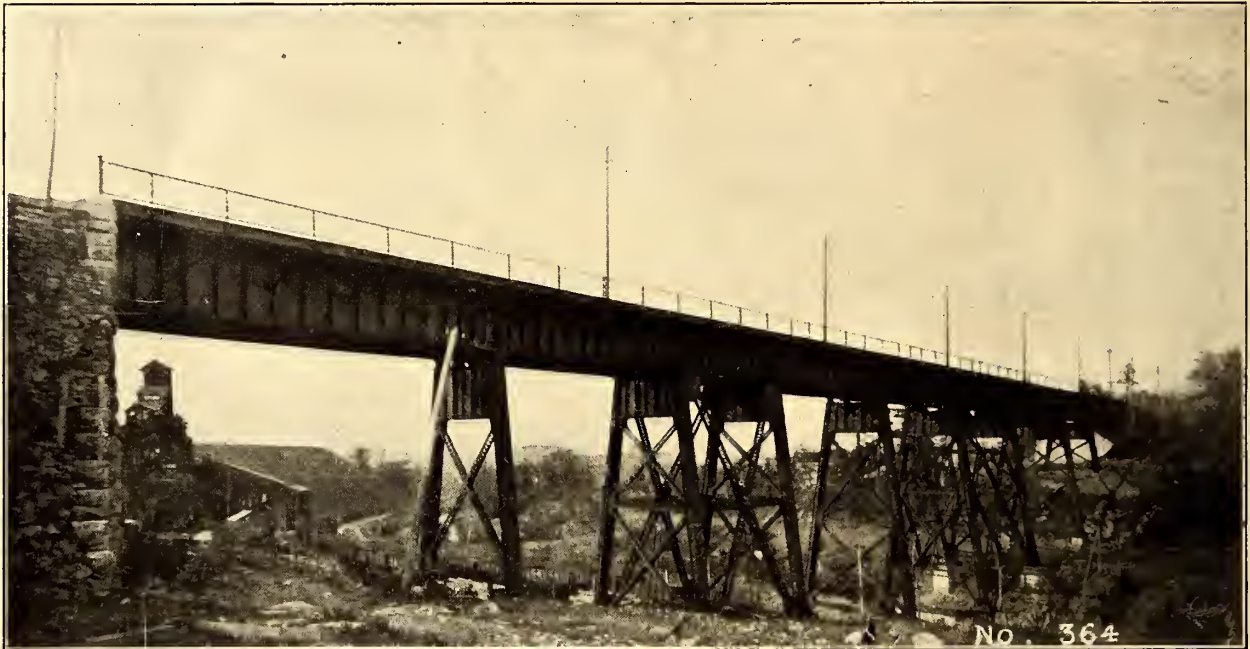
ONE OF THE VIADUCTS ON THE LINE
