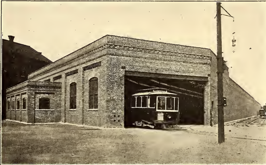
THE MAIN STREET, OR FRONT, END OF THE NEW CAR HOUSE
