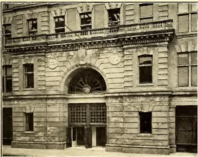
MAIN ENTRANCE TO THE BUILDING
