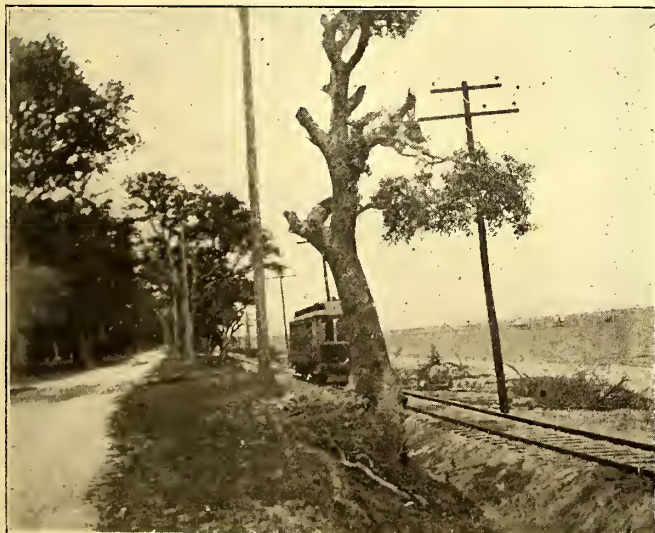
A VIEW ALONG THE LINE PARALLELING THE SHELL BEACH ROAD BETWEEN GULFPORT AND BILOXI
