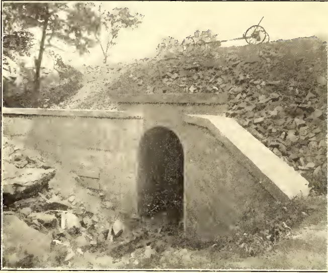
TYPICAL CONCRETE CULVERT
