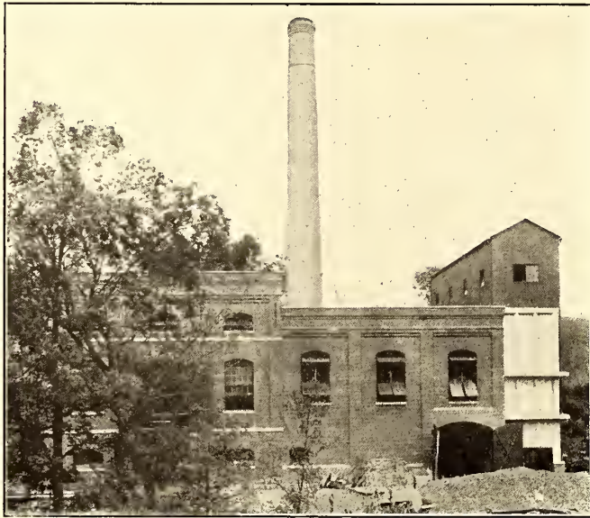
POWER STATION NO. 2 AT RIDLEY CREEK, SHOWING REINFORCED CONCRETE COAL BUNKER ON THE RIGHT
