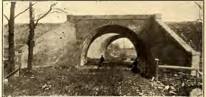
FIG. 7.—OVERHEAD CROSSING ON THE LIMA & TOLEDO RAILWAY
