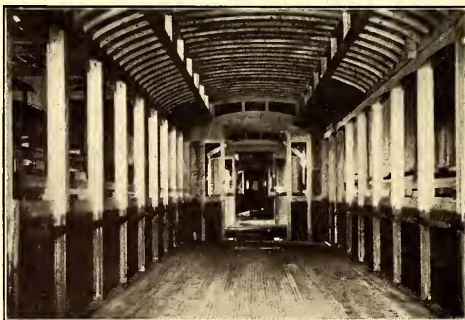
FIG. 8.—INTERIOR OF CAR UNDER CONSTRUCTION, SHOWING INSIDE TRUSSES
