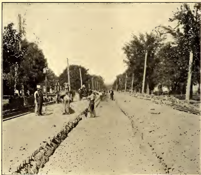
TRACK PARTLY LAID
