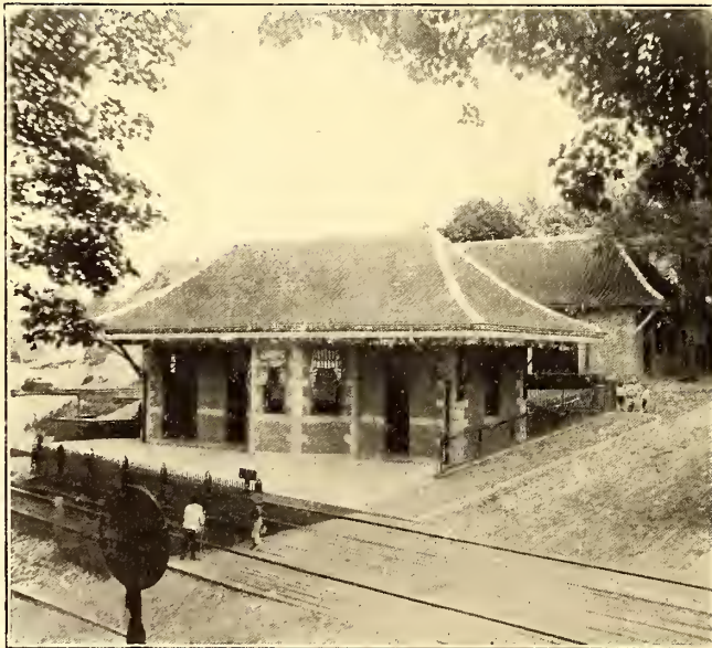
PITSTON PASSENGER STATION
