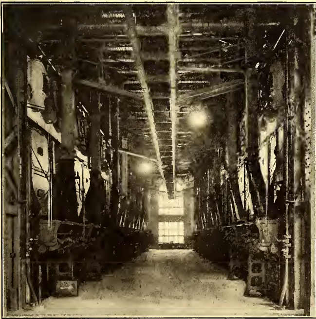
BOILER ROOM IN THE PORT MORRIS POWER HOUSE
