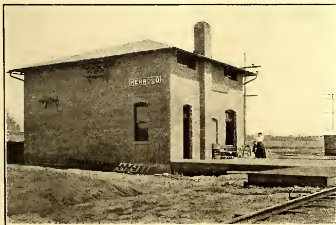
PRESENT SUB-STATION BUILDING AND STATION AT HERROLD
