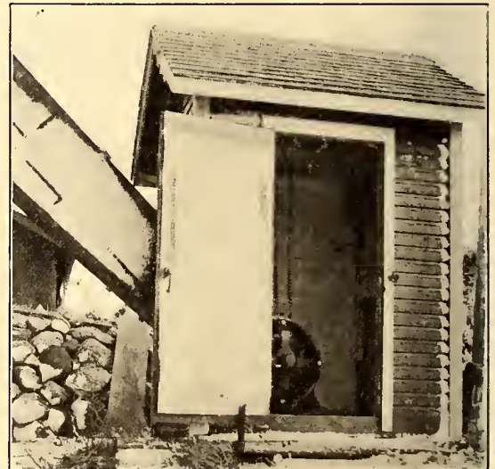
DETACHED MOTOR HOUSE, SHOWING CHUTE IN WHICH THE BELT IS CARRIED TO THE LINE SHAFT IN THE BARN
