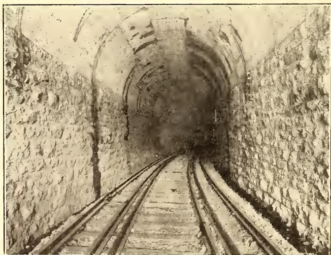
VIEW IN TUNNEL FROM NORTH PORTAL
