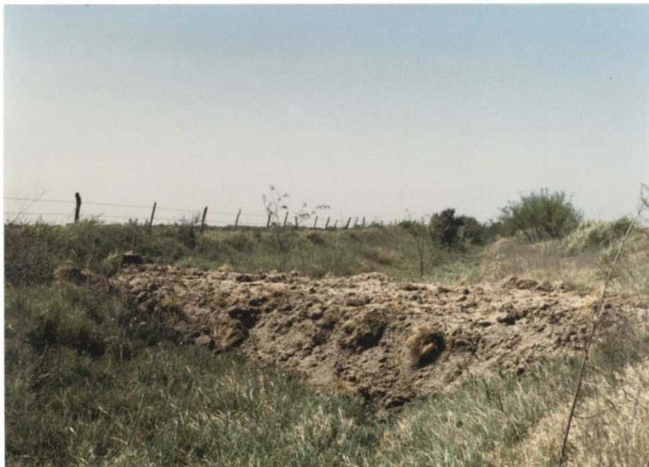
Drainage Ditches Plugged at Rudman Tract (4/86, N.M.G.)
