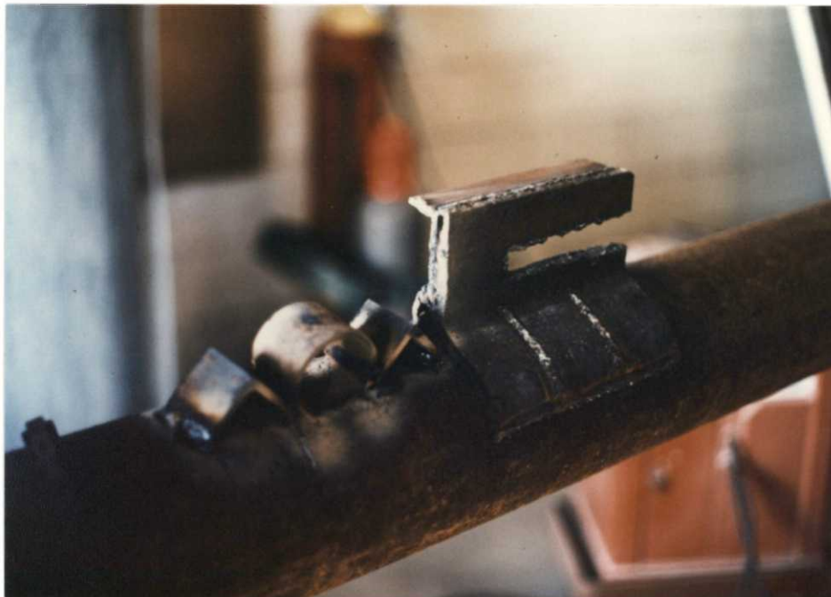
Modifications to the Cable Gate Chain Holding Mechanism Provides a Very Secure System (11/86, C.S.C.)
