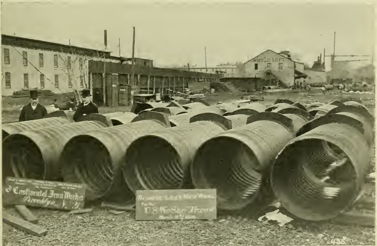
CORRUGATED FLUES FOR BATTLESHIP "TEXAS," MADE BY THE CONTINENTAL IRON WORKS BROOKLYN N. Y.
