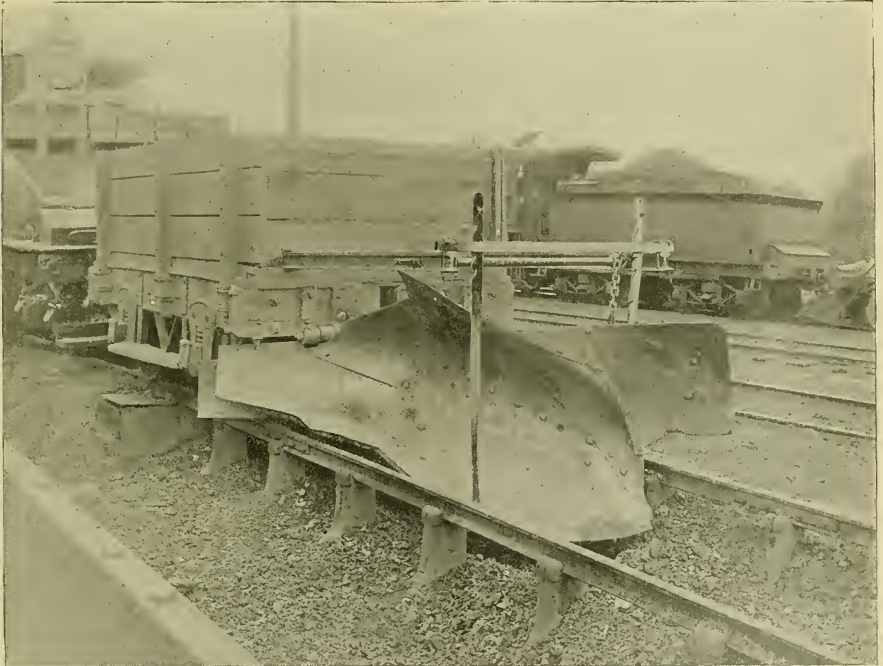
PLOW FOR CLEARING CINDER PITS, NEW YORK, LAKE ERIE AND WESTERN RAILROAD.
