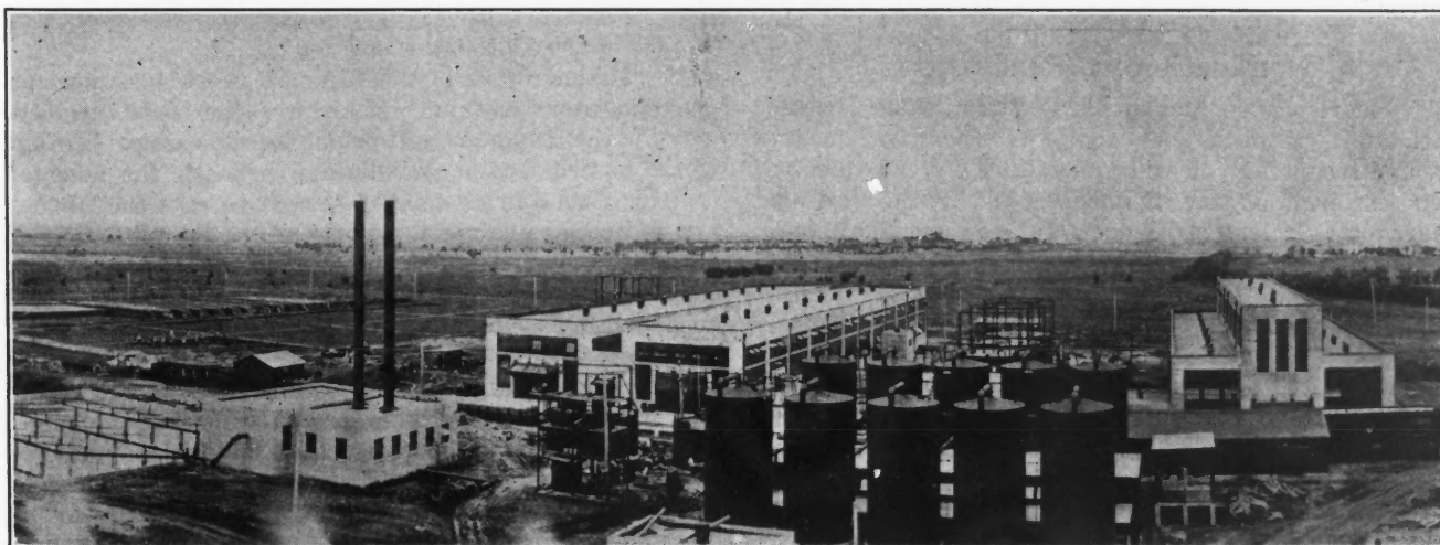
HELIUM PRODUCTION PLANT, FORT WORTH, TEX.
