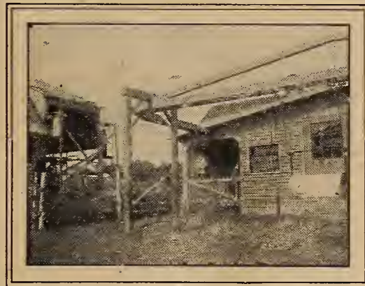
Corner of Beyer dairy barn, showing overhead carrier and track
