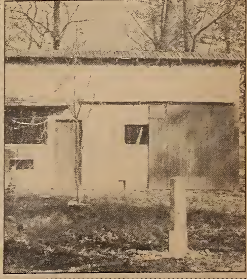
Concrete hitching-post and wagon-shed
