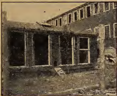
The paper house—good even in cold climates. In summer all the windows are removed
