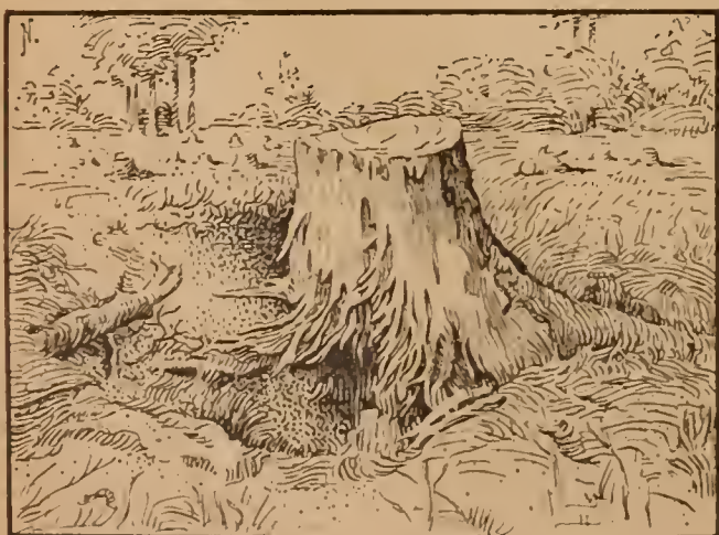
Effect of a charge placed too shallow; a large hole torn in the ground is the result
