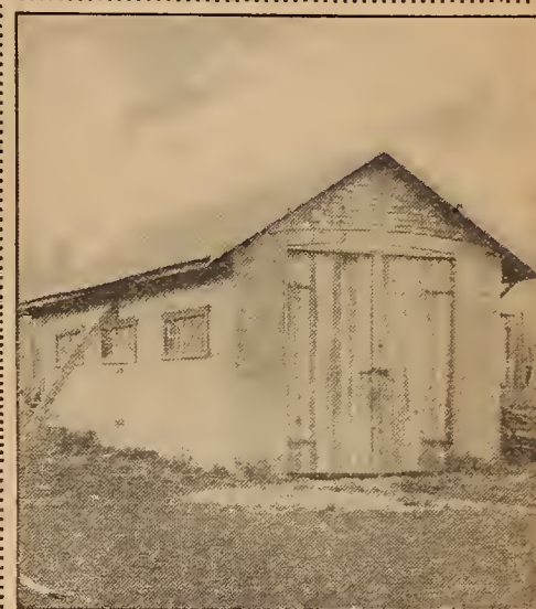
A fire-proof concrete engine-house
