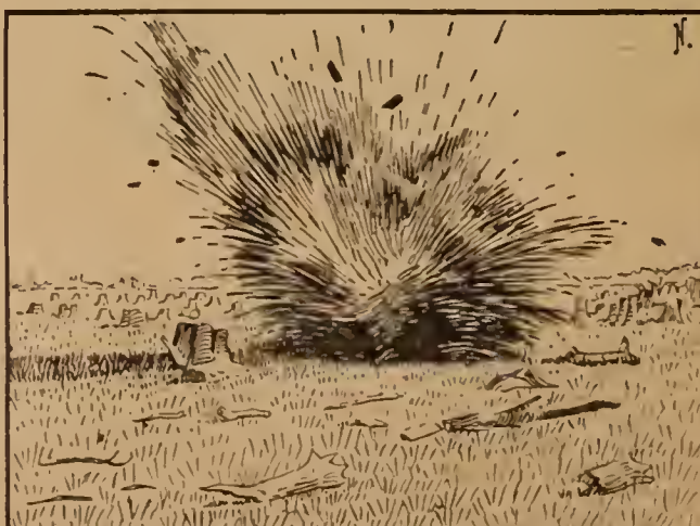
Effect of a charge correctly placed; the stump is shattered and completely removed
