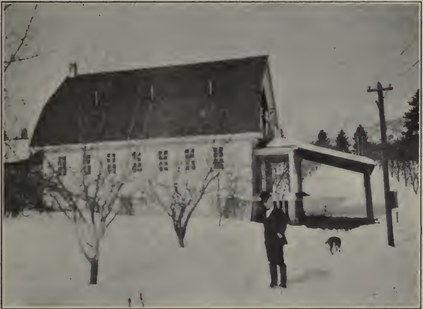
Fig. 10. Fruit storage and packing house of Capt. R. J. Graham, Cashmere, Wash. Note the ventilator-stacks along the roof.
