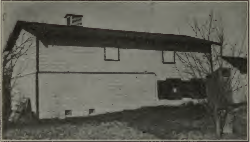
Fig. 4. A British Columbia fruit-storage house built by Thos. Brydon, Royal Oak, V.I. It has often saved its cost by holding fruit to suit the demands of local markets in Victoria. Note the ventilators at the base of the building to admit the cold night air.
