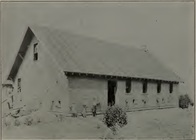
Fig. 5. A Wenatchee Valley fruit storage built by Dr. Whitney, of Cashmere, Wash. Note the ventilating system.
