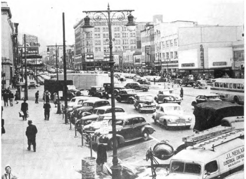
This street is U S Route 422 in Reading, Pa. Its extreme width is negated by the lack of channelization or control, as evidenced by the haphazard, crowded vehicular movements.
