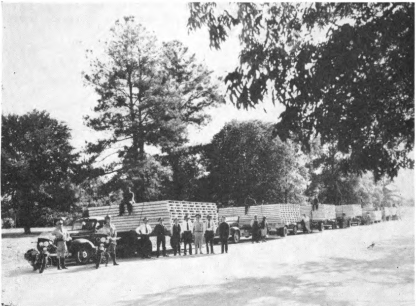
Access roads are an important adjunct to military establishments. This truck fleet of tent platforms was on the way to Camp Shelby, Miss., where a tent city was built to quarter 50,000 soldiers in training.
