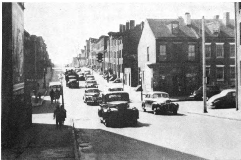
This is one of a pair of one-way streets that carry U S Route 40 through Baltimore, Md. Note the different widths of pavement in the two blocks. A stopgap, relatively unsatisfactory means of handling heavy city traffic, there are 695 miles of such pairs of one-way streets on the interstate system.
