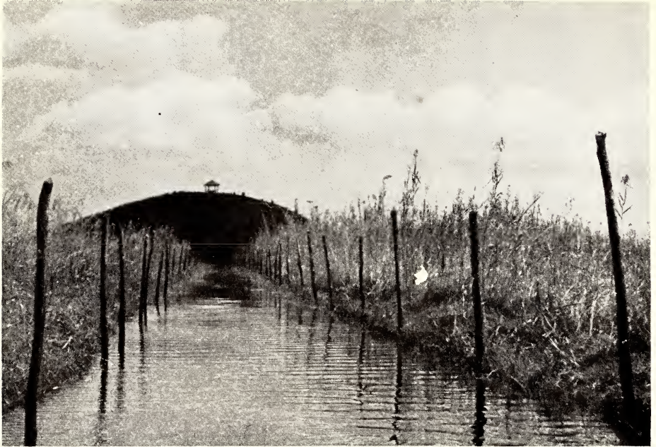
Canal with observation hillock and tower
