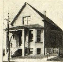
A No. 2118 IDEAL Boiler and 270 ft. of 38-in. AMERICAN Radiators, costing owner $135, were used to Hot-Water heat this cottage.
