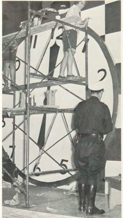
a ticket for parking a scaffold?
