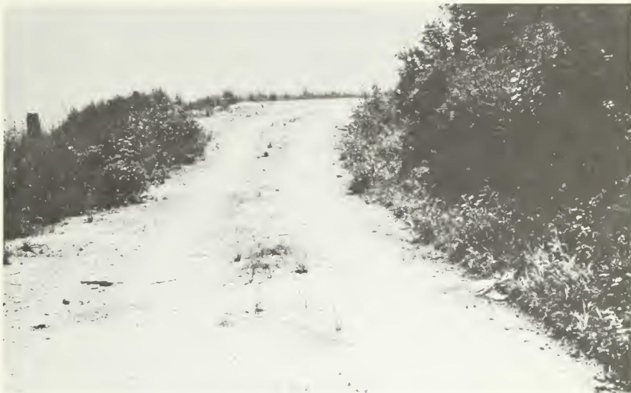
Figure 6.--Break in grade, with dip followed by turnout on outslope section.
