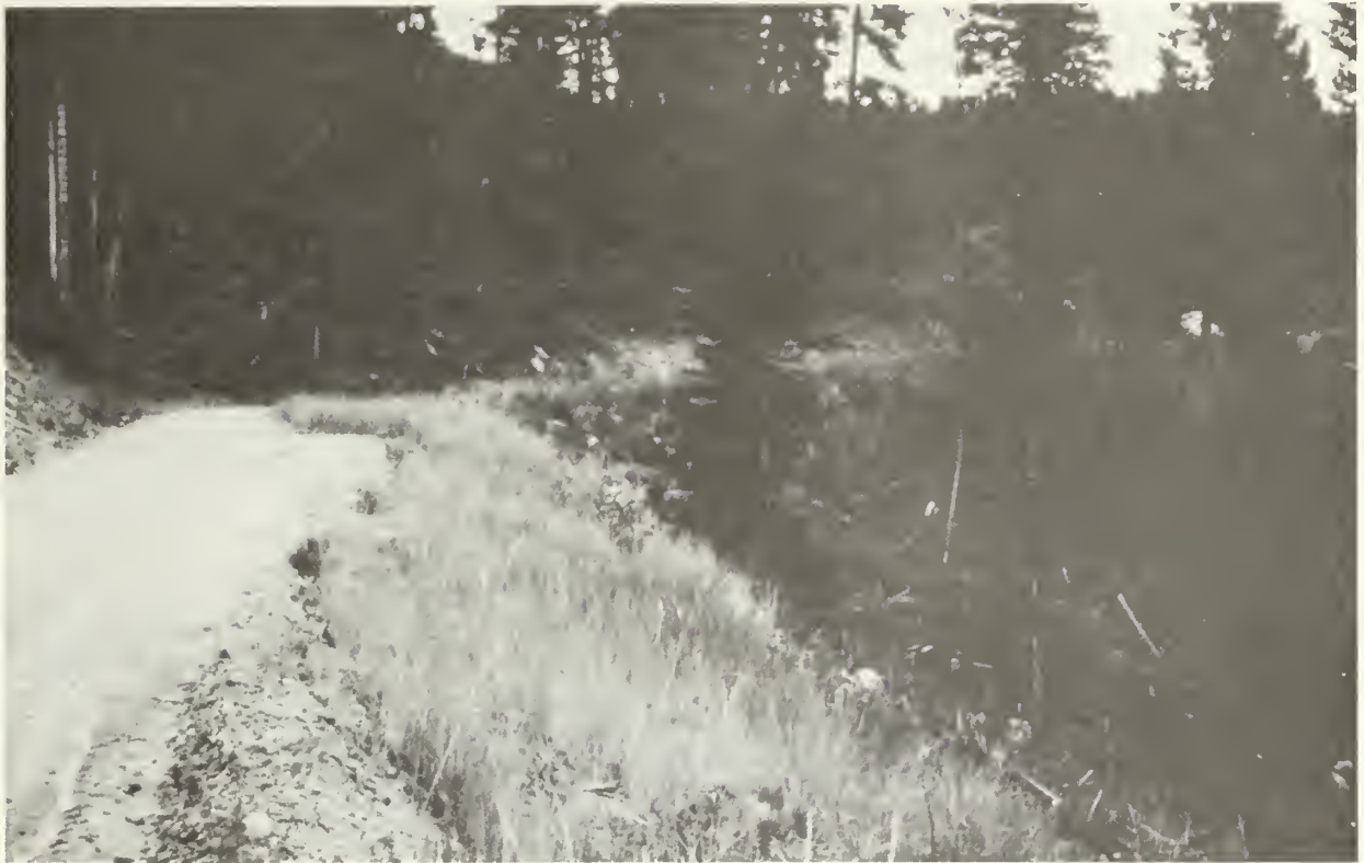
Figure 9.--Typical section of stable, sidecast fill.
