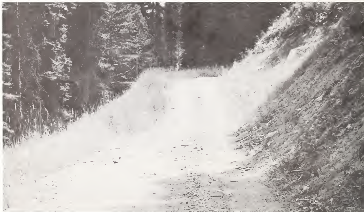
Figure 5.--Outsloped section with dip (built after construction).
