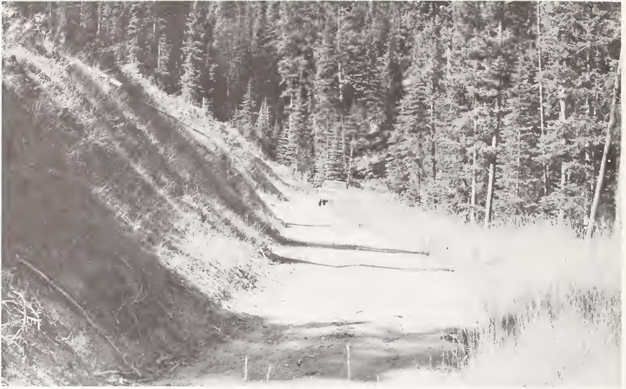
Figure 11.--Revegetation of cut-and-fill slopes.
