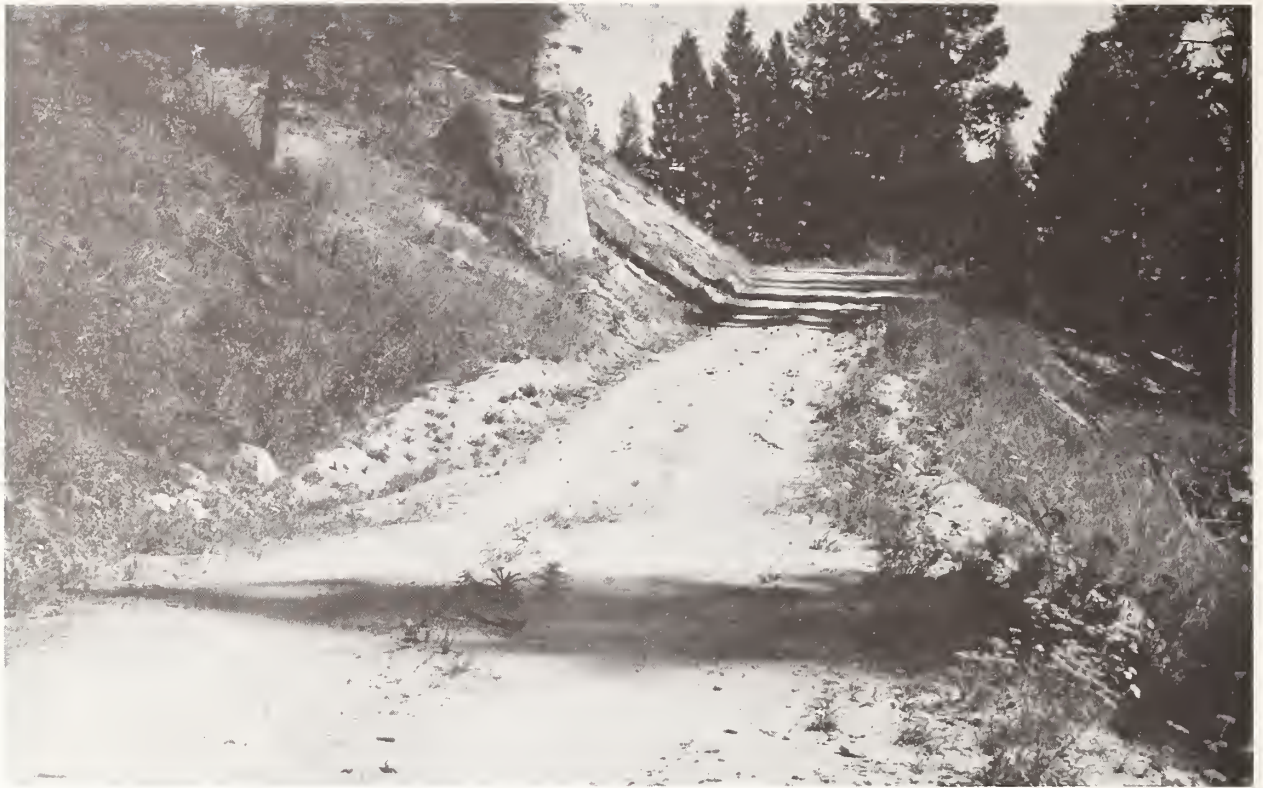
Figure 8.--Insloping to dip with berms controlling flow.
