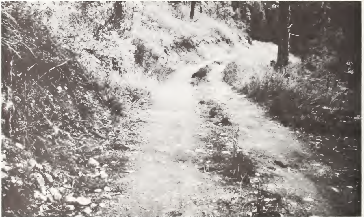
Figure 15.--Short, stable vertical backslopes on uniformly sloping terrain.
