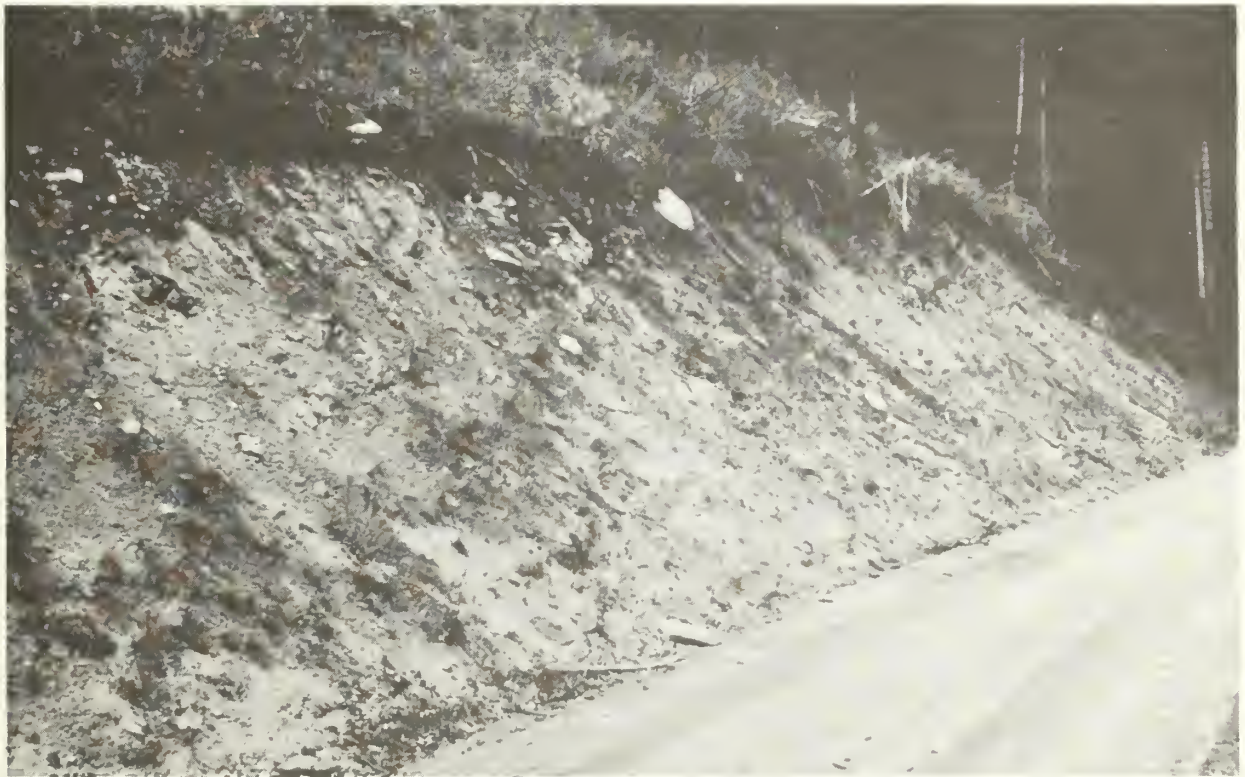
Figure 10.--Typical section of stable 1:1 cut slope.
