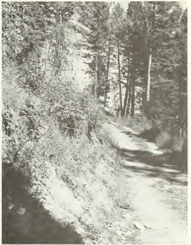
Figure 16.--Transition from 3/4:1 to vertical backslopes going away from the camera.
