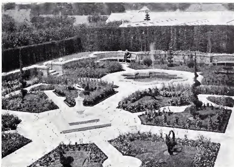
DUTCH GARDEN AT "WEST HALL," BYFLEET DESIGNED BY G. LISTER SUTCLIFFE, ARCHITECT
