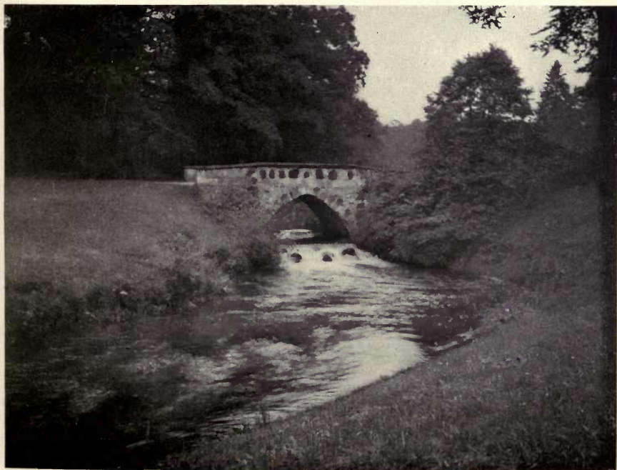
A Rough Stone Bridge in the Park on the Estate of Prince Pückler von Muskau.
