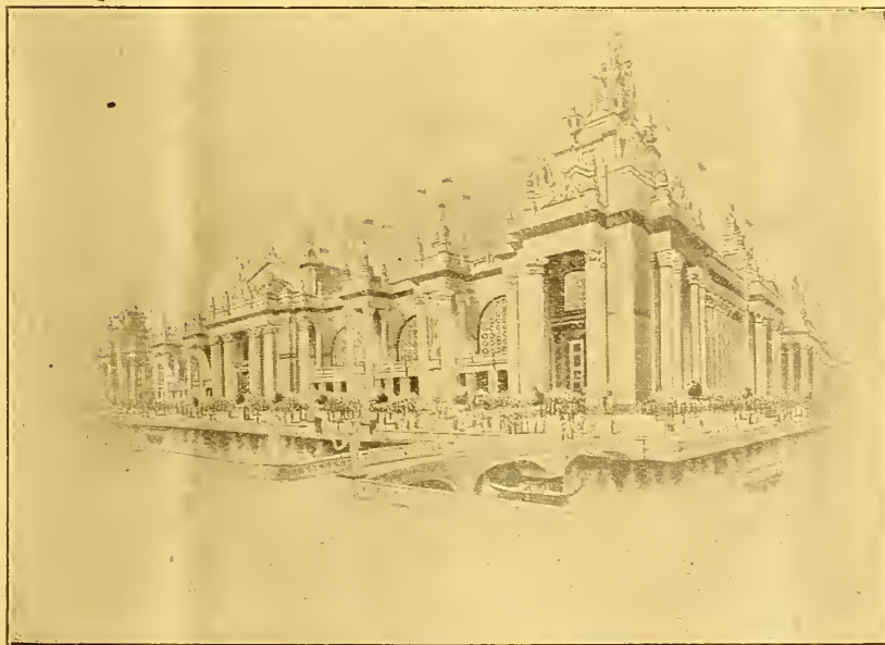
Electricity Building, World's Fair, St. Louis. See page 2.
