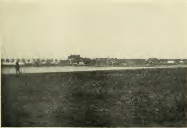
SANDING THE CLEARED PEAT GROUND FOR FARMING
