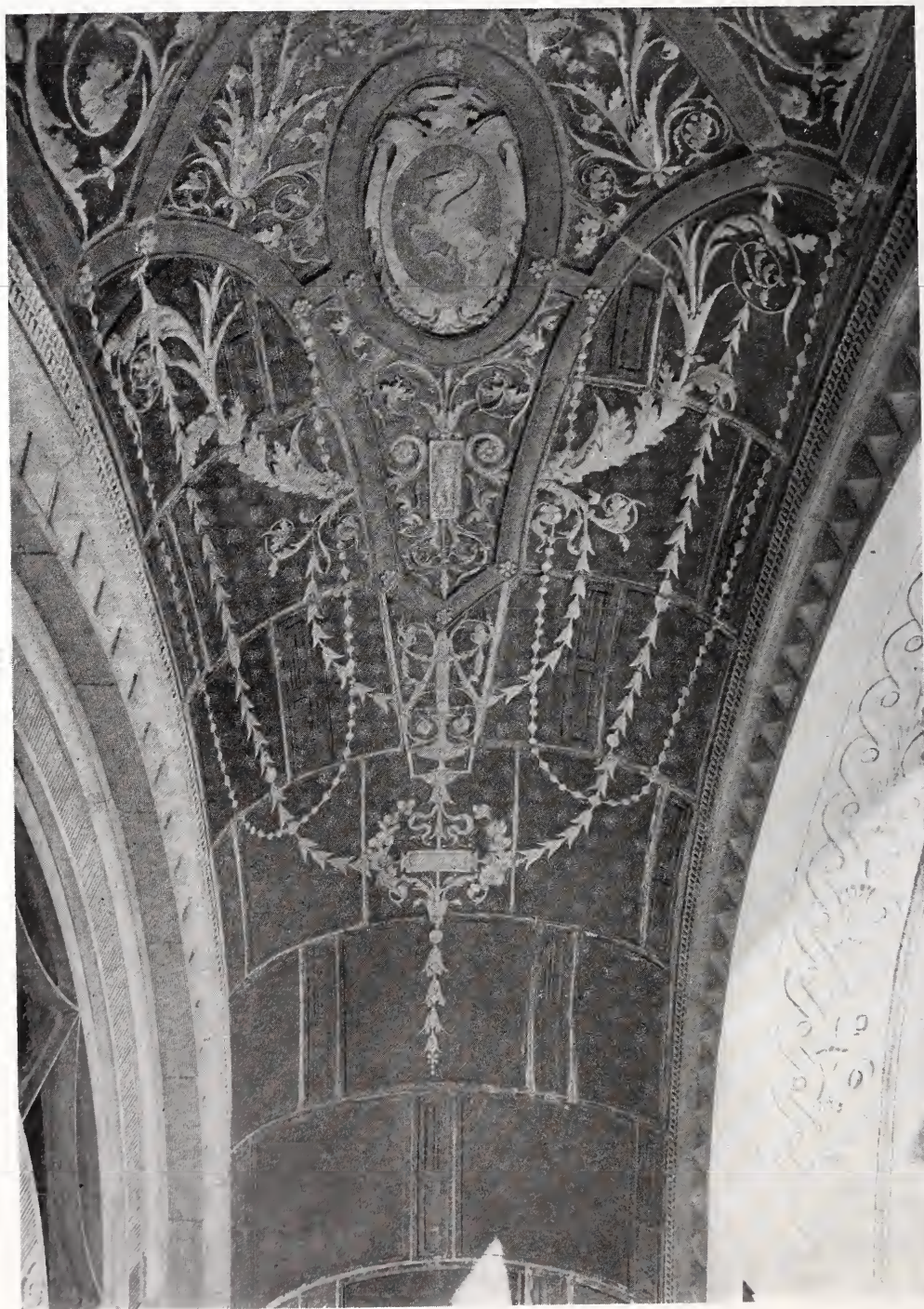
DETAIL OF CEILING IN MAIN ENTRANCE—HADDINGTON BRANCH OF THE FREE LIBRARY OF PHILADELPHIA. ALBERT KELSEY, ARCHITECT.
