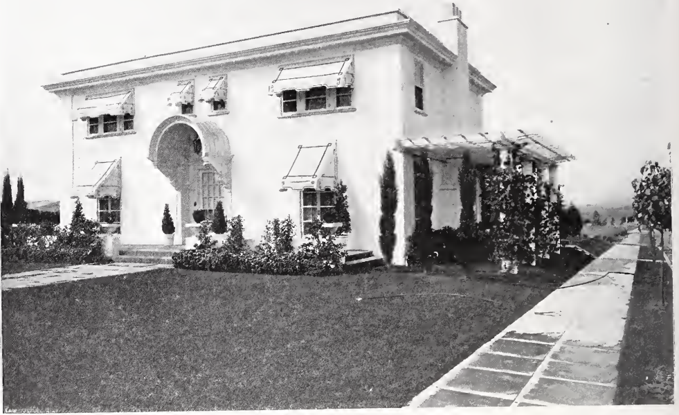
HOUSE OF CHARLES AMILLO, ESQ., LOS ANGELES, CAL. B. Cooper Corbett, Architect.
