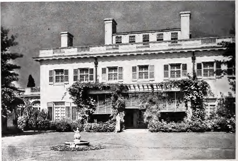
GARDEN FRONT—HOUSE OF EDWARD COYKENDAL, ESQ., KINGSTON, N. Y. York & Sawyer, Architects.
