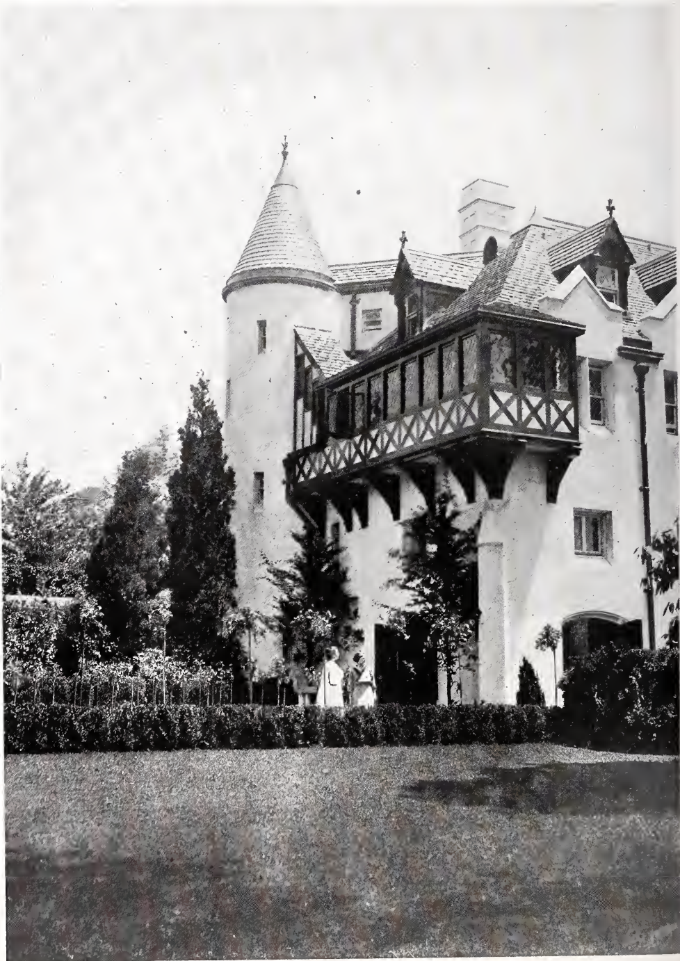
END ELEVATION—RESIDENCE OF MRS. FLORENCE H. MARJON, SHIPPAN POINT, STAMFORD, CONN. HUNT & HUNT, ARCHITECTS.
