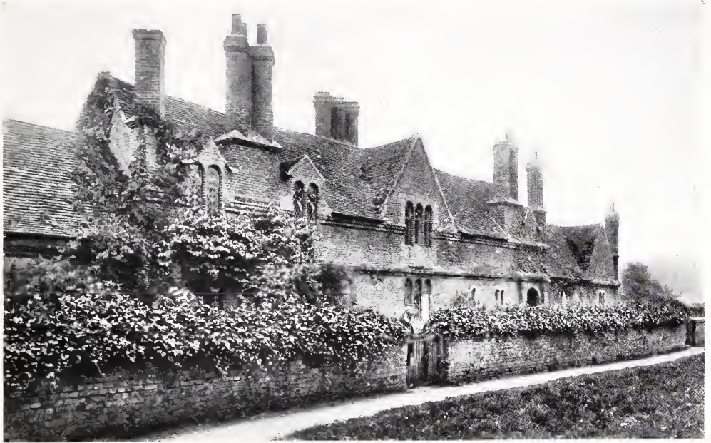
THE "ABBNEY," AT AUDLEY END, STAFFORDSHIRE, WITH SKETCH PLANS SHOWING POSSIBLE LAYOUT OF FLOORS.
