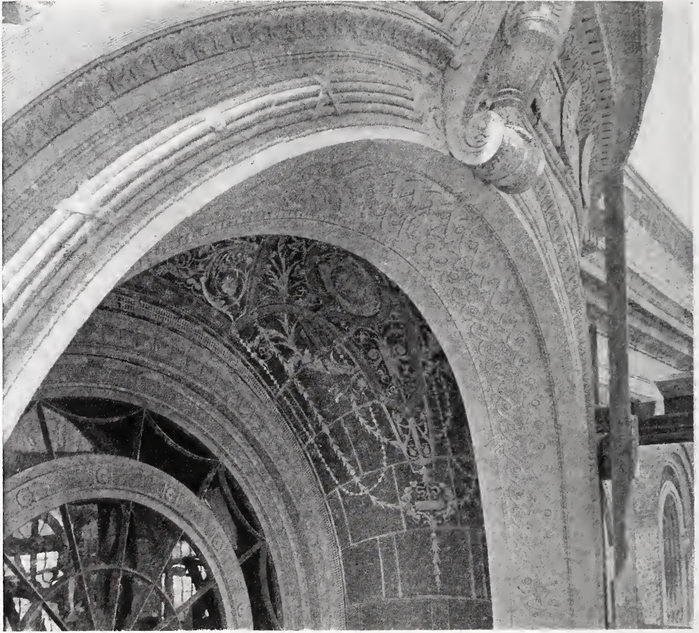
ARCH OVER MAIN ENTRANCE—HADDINGTON BRANCH OF THE FREE LIBRARY OF PHILADELPHIA.
