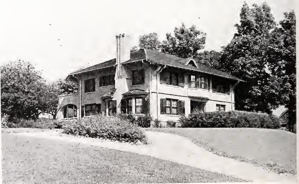
FIG. 26. HOUSE OF DEAN H. M. BATES, ANN ARBOR, MICH. Samuel McC. Stanton, Architect.
