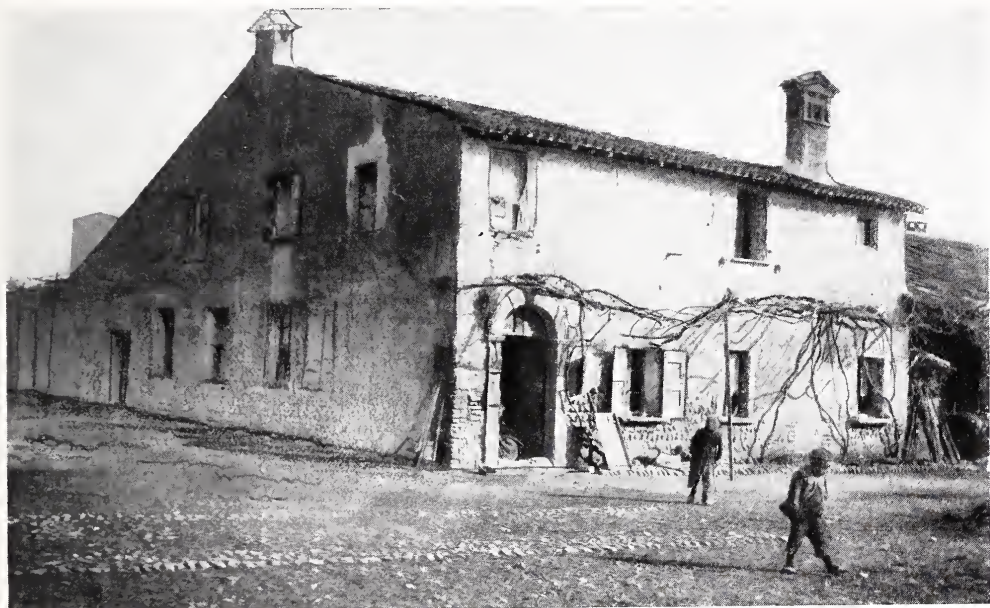
ITALIAN HOUSE ON THE STRADA CHIODA, NEAR VERONA. WITH SKETCH PLANS SHOWING POSSIBLE LAYOUT OF FLOORS.
