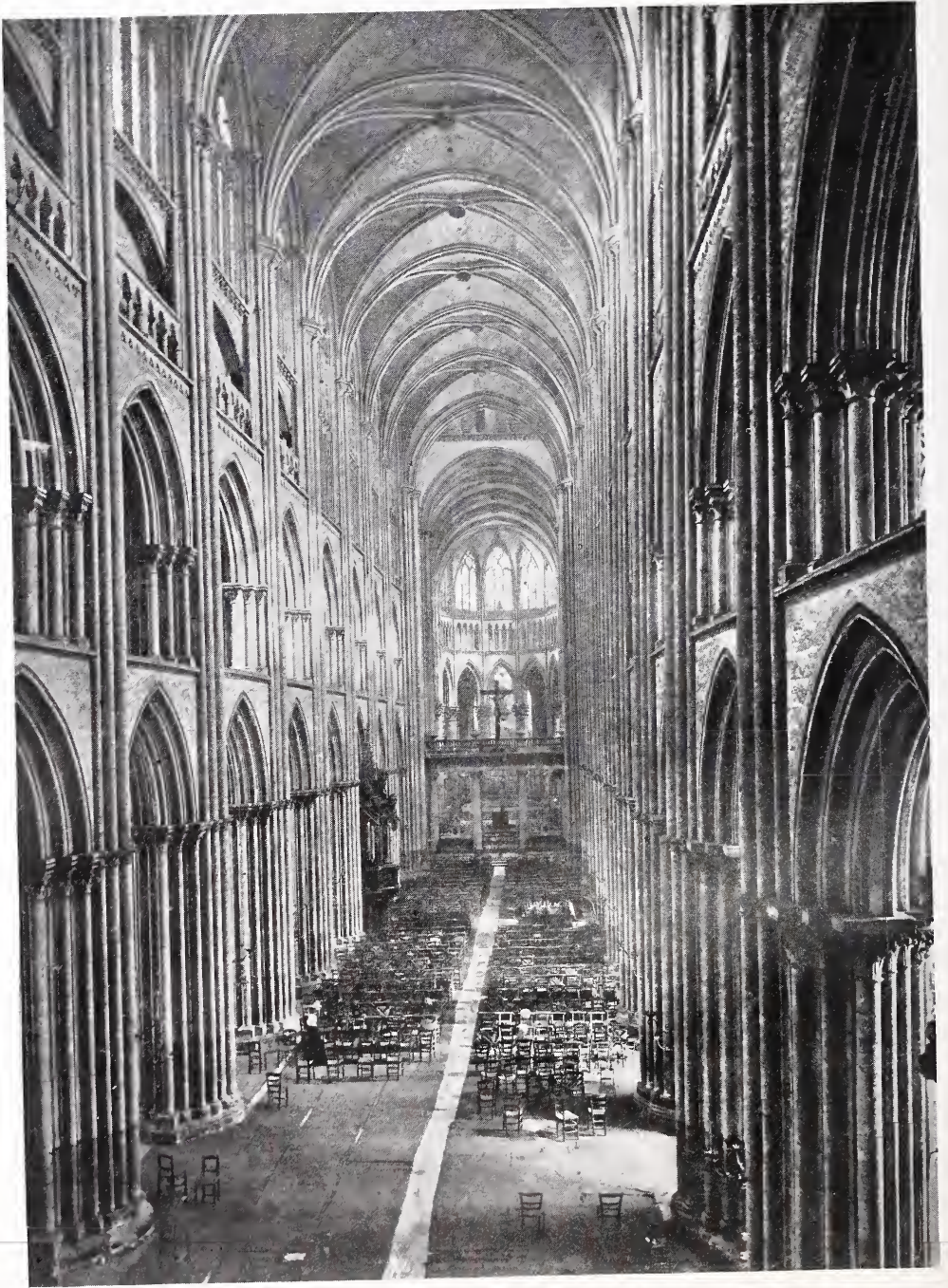
FIG. 3. NAVE OF ROUEN CATHEDRAL. RIBBED VAULTING AND VAULTING SHAFTS.
