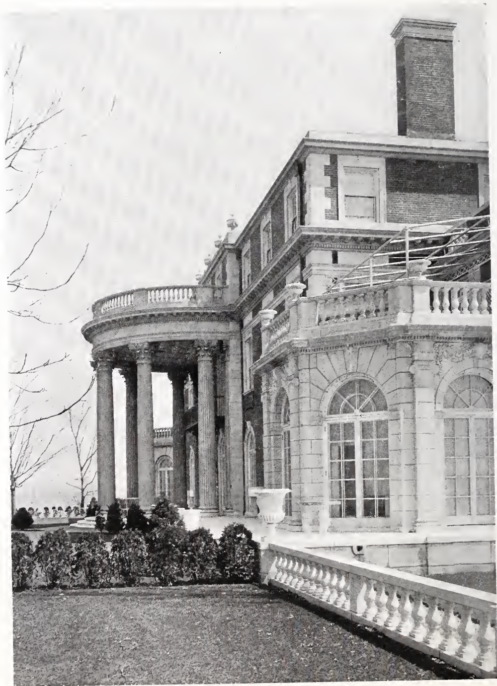
NORTH ELEVATION—COUNTRY HOUSE OF ORMOND G. SMITH, ESQ., OYSTER BAY, L. I. HOPPIN & KOEN, ARCHITECTS.
