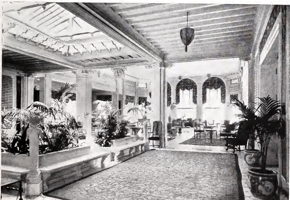
FIG. 10. FOUNTAIN COURT AND SOLARIUM, LOOKING EAST—SOUTH SHORE COUNTRY CLUB, CHICAGO. Marshall & Fox, Architects.
