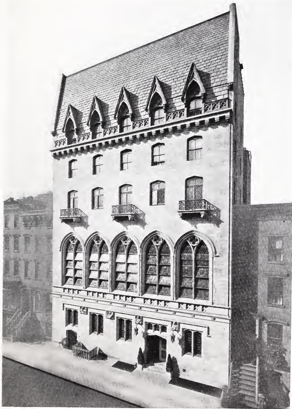
THE FRIARS CLUB, NEW YORK. HARRY ALLAN JACOBS, ARCHITECT.
