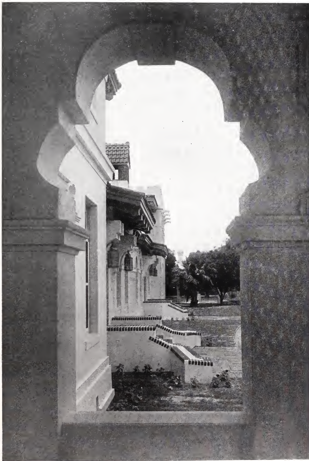
VIEW FROM PORCH BAY—SANTA GERTRUDIS RANCH HOUSE, THE HOME OF MRS. H. M. KING, NEAR KINGSVILLE, TEXAS. ADAMS & ADAMS, ARCHITECTS.
