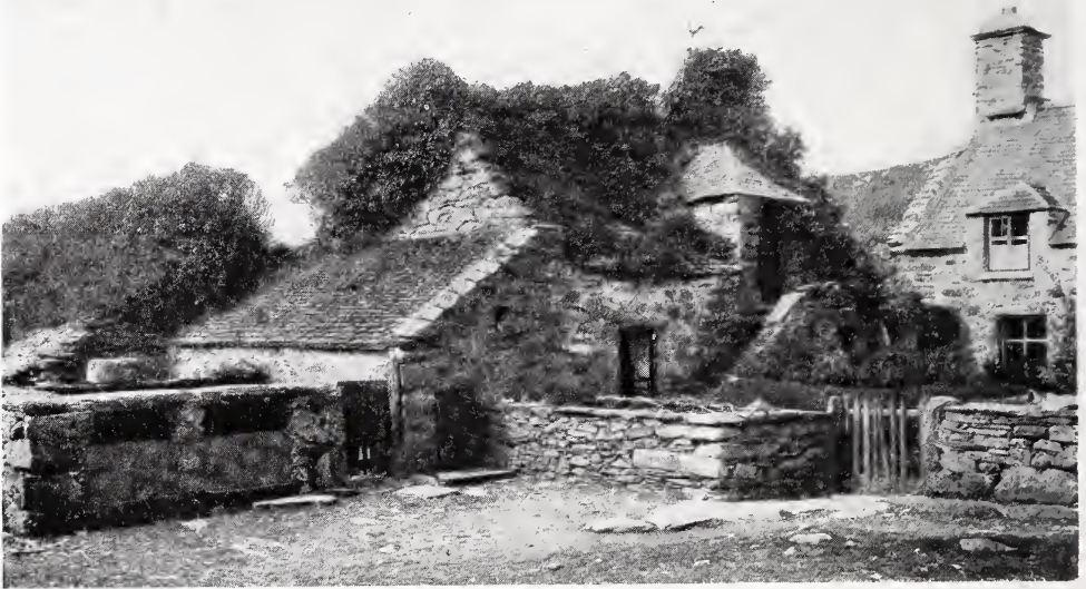
STONE FARMHOUSE, ON A HILLSIDE AT BARMOUTH, WALES, WITH SKETCH PLANS SHOWING POSSIBLE LAYOUT OF FLOORS.
