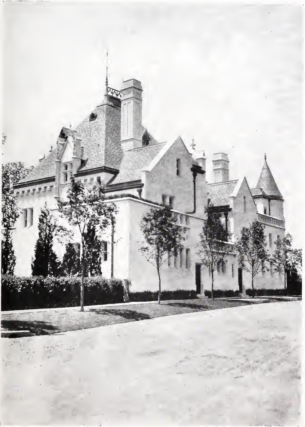
ENTRANCE FRONT—RESIDENCE OF MRS. FLORENCE H. MARION, SHIPPAN POINT, STAMFORD, CONN. HUNT & HUNT, ARCHITECTS.
