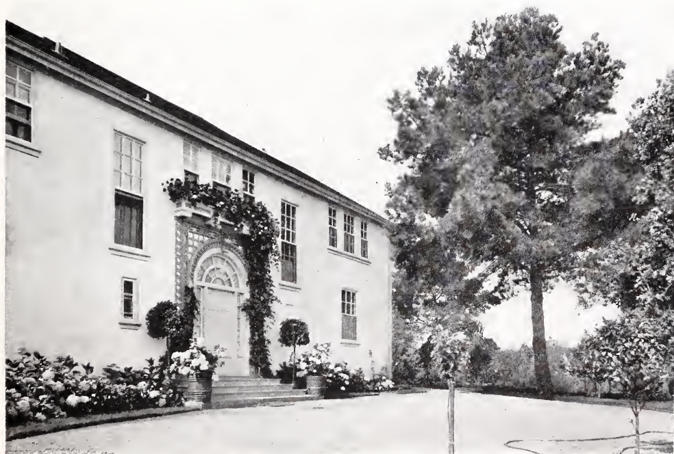
ENTRANCE DETAIL—HOUSE OF DR. W. C. CHIDESTER. Lewis P. Hobart, Architect.
