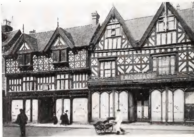
STREET FRONTS OF TWO BUILDINGS, CHESTER, ENGLAND.
