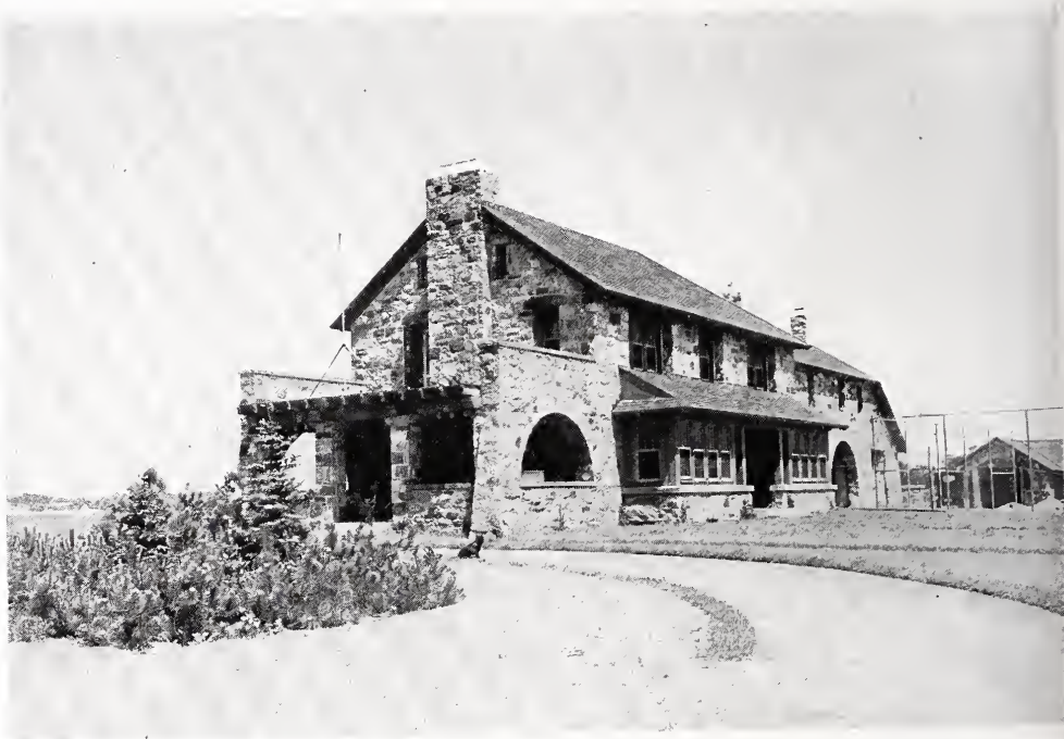
RESIDENCE OF THOMAS ROBINS, ESQ., SHIPPAN POINT, STAMFORD, CONN. Hunt & Hunt, Architects.
