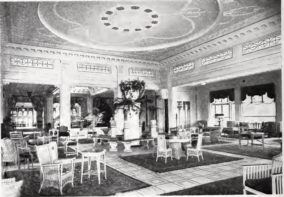
FIG. 11. SOLARIUM, LOOKING N.W.—SOUTH SHORE COUNTRY CLUB, CHICAGO. Marshall & Fox, Architects.
