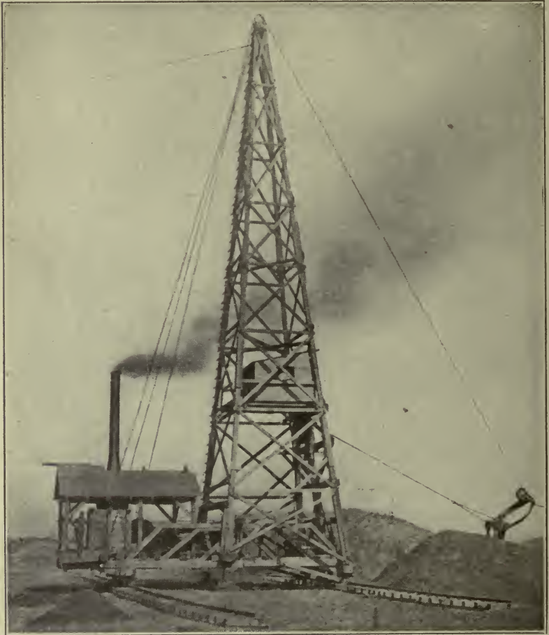
Fig. 39. Tower Excavator Operating on New York State Barge Canal
