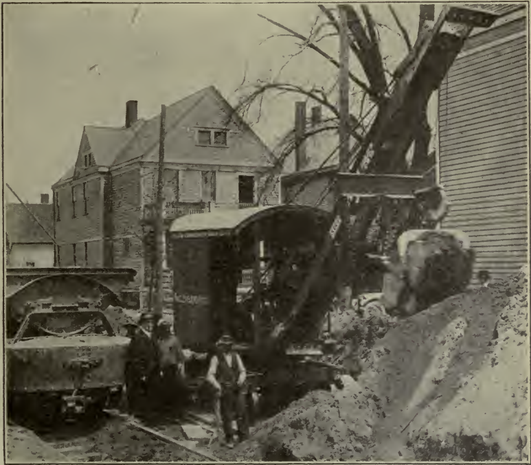
Fig. 24. Electrically Operated Power Shovel
