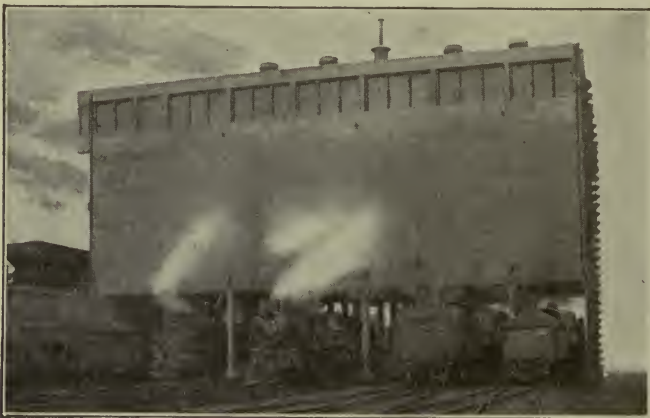
Fig. 78. Electrically Operated 2000-Ton Coaling Station Fourteen engines can be supplied simultaneously with coal, sand, and water. Courtesy of Link-Belt Company, Chicago
