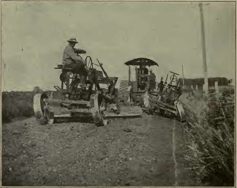
●Fig. 8. Scraping Grader Especially Designed for Constructing Ditches
