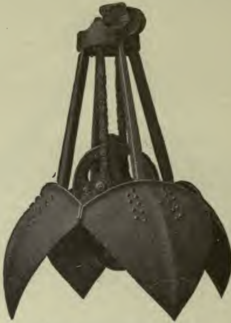
Fig. 49. Typical Orange-Peel Bucket Courtesy of The Hayward Company, New York City
