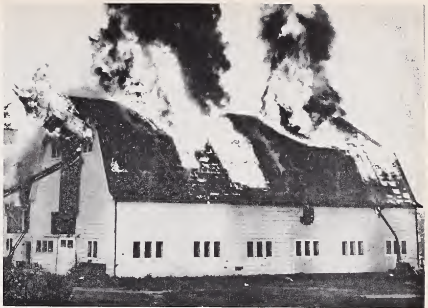
Typical dairy barn fire involving hay loft.
