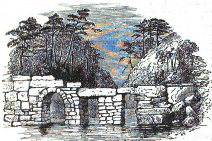
OLD BRIDGE AT AMWEE.
