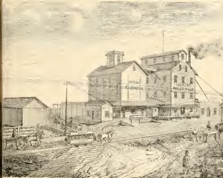
CRESCENT MILLS AND ELEVATOR, EAU CLAIRE.
