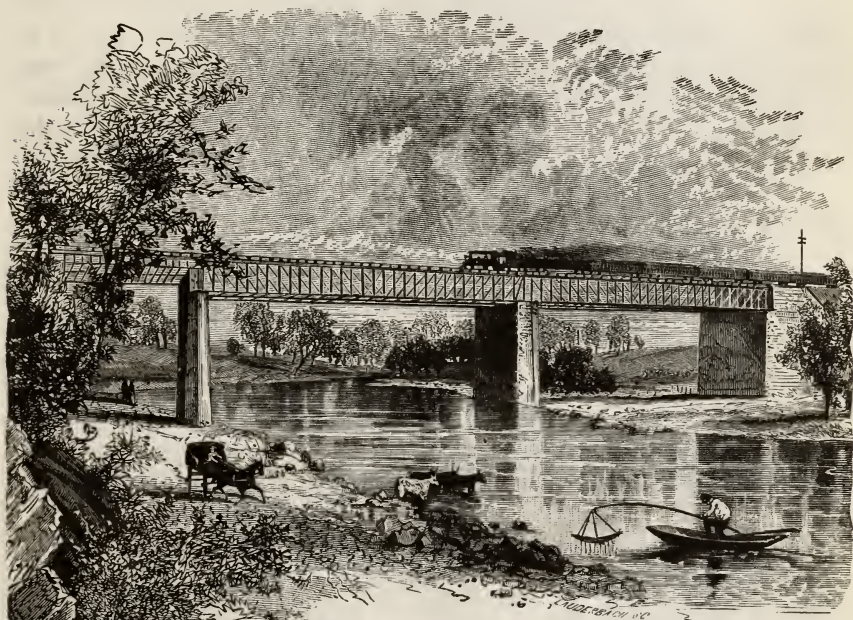
BRIDGE. — CONESTOGA RIVER.
