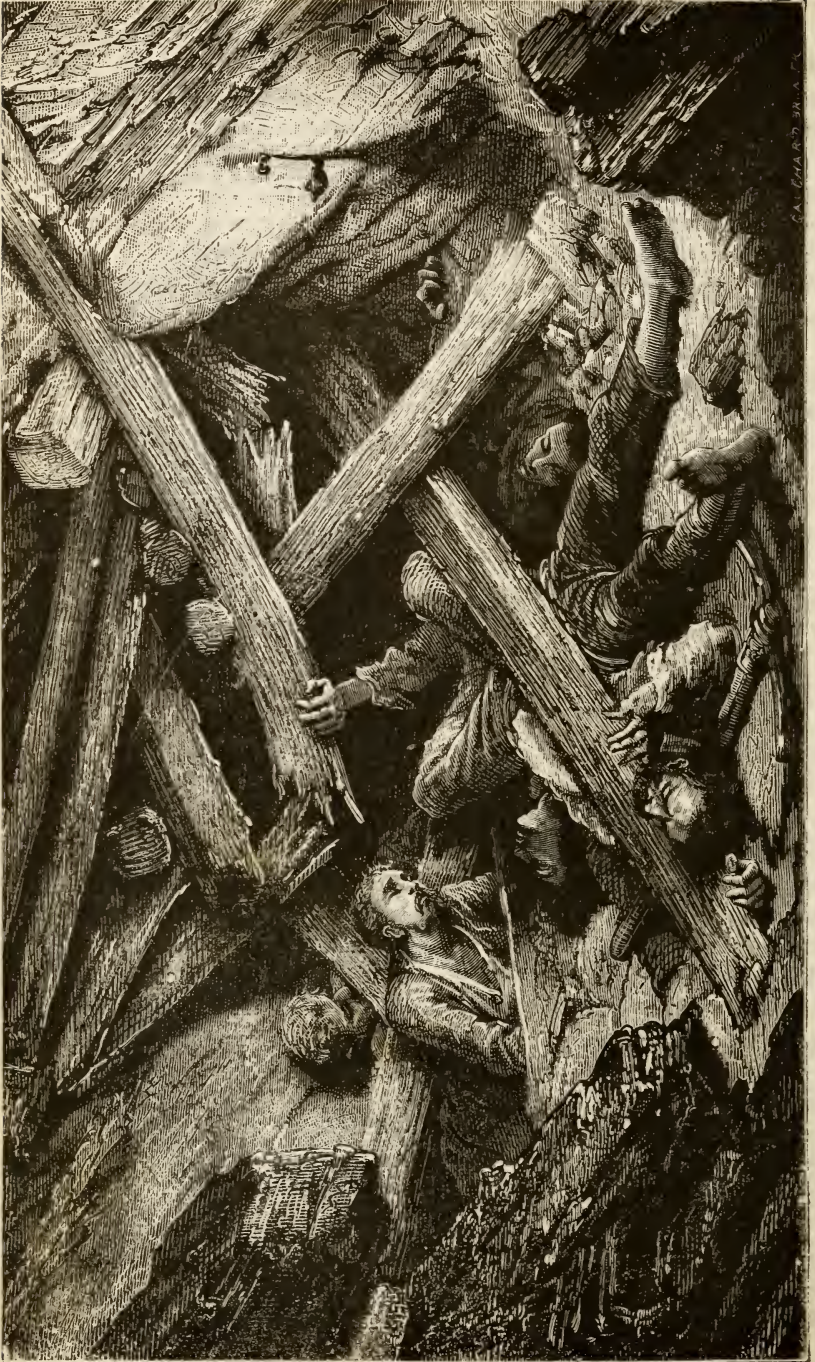
FALLING-IN OF A MINE.
