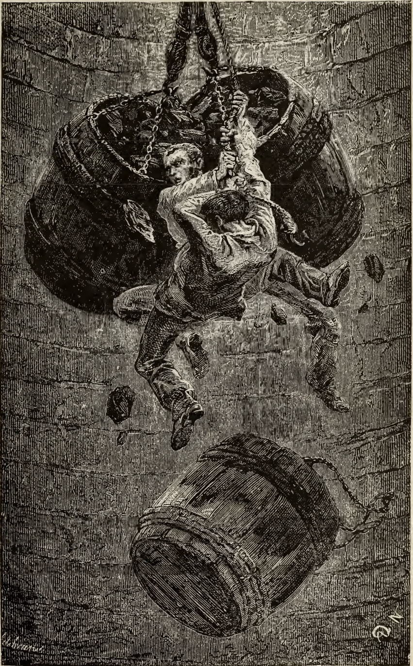
COLLISION OF TUBS IN A SHAFT.
