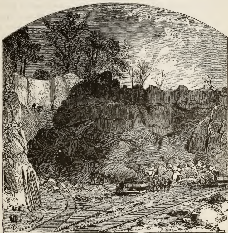
CUT IN IRON MOUNTAIN.
