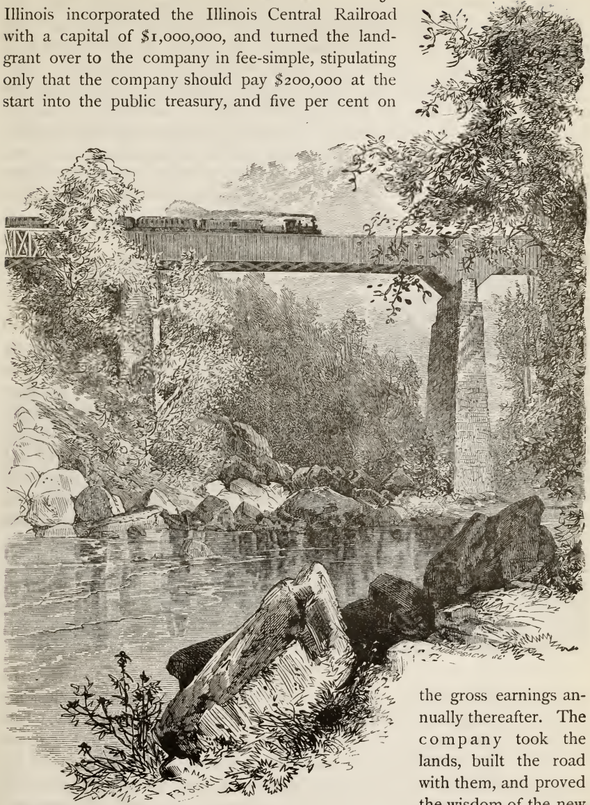
BRIDGE. — CONEWAGO CREEK.
