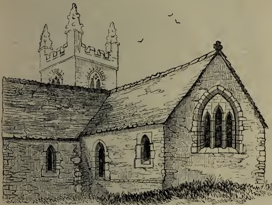
South-east View of Chancel and Transept, Manaccan.
