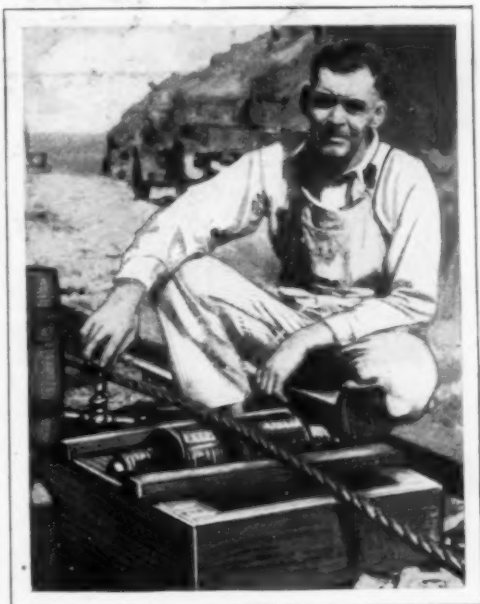
Automatic Oiling Unit to Keep Cables in Good Condition and Prolong Their Life
