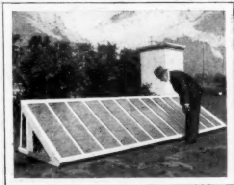
Water-Heating Plant That Utilizes the Sun; the Storage Tank Is Seen in Background at Right
