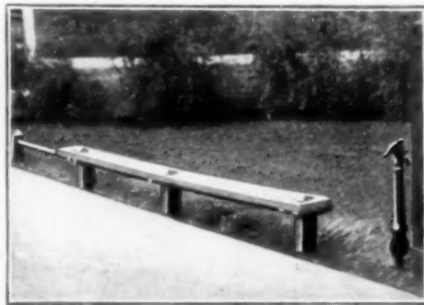
Simple Seat on Filling-Station Guardrail Can Be Made from a Plank
