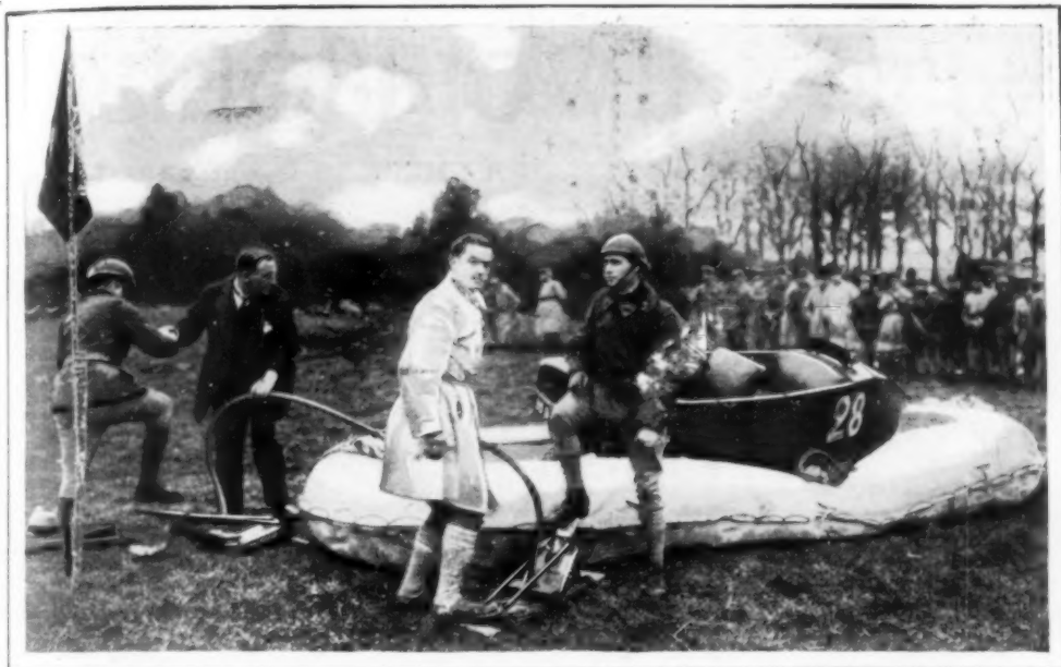
Blowing Up the Rubber Boat to Give the Motorcycle a Ride; the Collapsible Floats Have Been Found Increasingly Useful in the French Army, Where Special Development of the Motorcycle Is under Way
