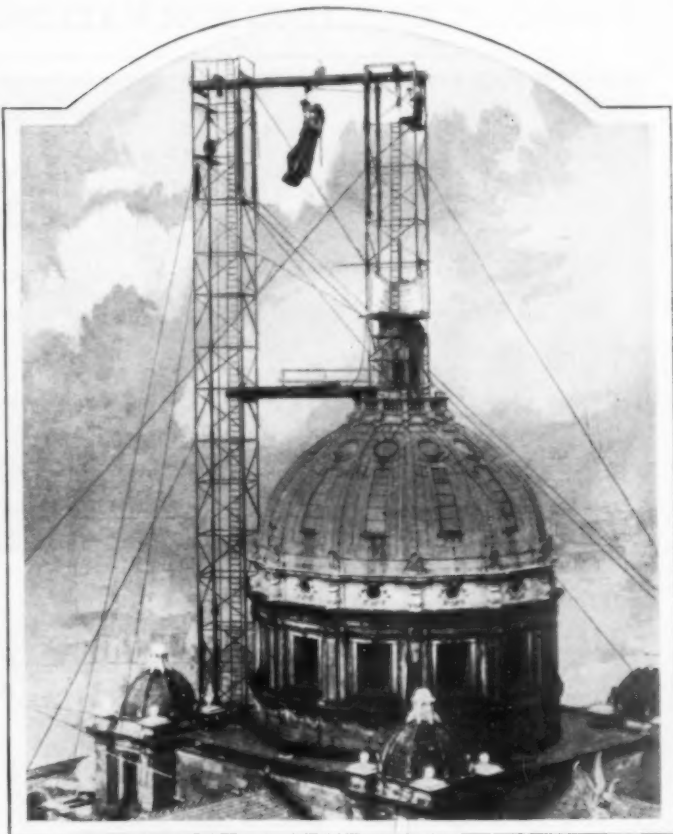
Huge Statue of Washington Being Erected on Courthouse Dome; Pulling the Figure Across Preparatory to Lowering
