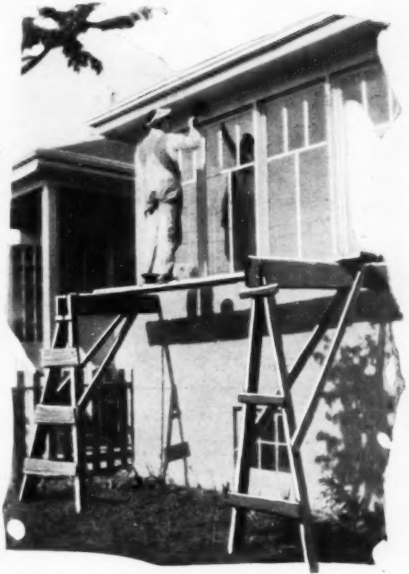
Simple Lean-To Scaffold Is Easy to Erect and Takes Little Space in the Workman's Truck
