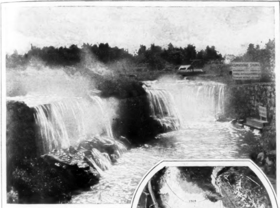
Miniature Niagara Falls Built to Study Conservation Problem, and Aerial Photo of Horseshoe Falls, Showing Crest Lines of Past Years
