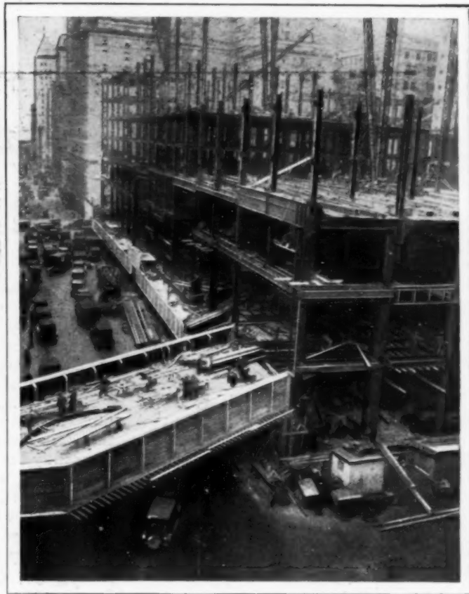
Where Autos Will Pass through a Skyscraper; One of the Drives That Leads into the Huge Building as It Appeared under Construction
