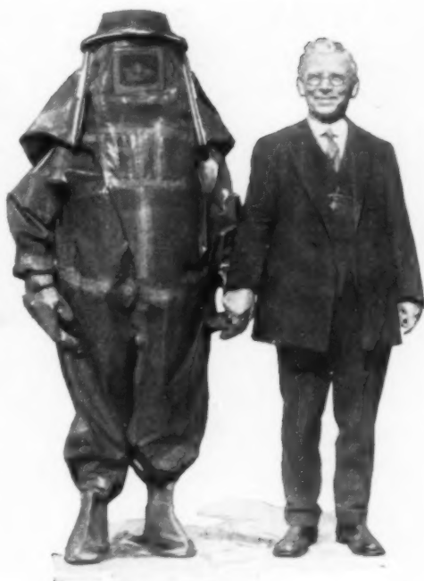
Life-Saving Suit That Weighs but Twenty-One Pounds and Has Pockets Inside to Hold Food and Water
