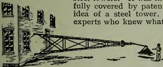
Testing the Towers.
