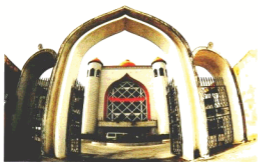
百崎回族乡政府大楼 Huizu Village Government Building in Baiqi
