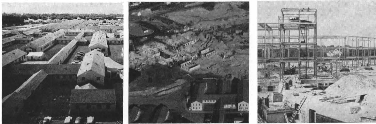
THE "BEFORE, DURING AND AFTER" STAGES in the development of the present Administration Building are (above from left to right) the old Administration Building, the partly completed foundation of the new building and the structure's bare steel framework. Below (left to right) is the building nearing completion, the laying of the cornerstone by Rear Admiral Walter S. DeLany, then Commandant of the Third Naval District, and the Administration Building as it is today.
