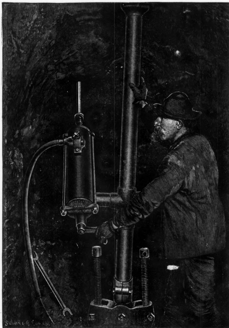
EDISON ELECTRIC PERCUSSION DRILL, LAST CHANCE MINE, WARDNER, IDAHO.
