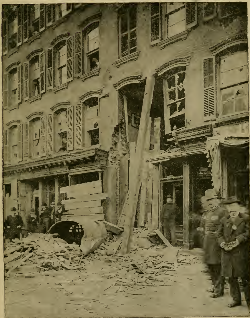
FIG. 2. — SHOWING THE DAMAGE DONE BY THE FRONT HEAD.
