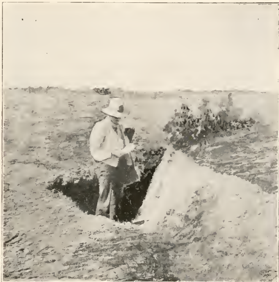
SPANISH TRENCH IN FRONT OF BLOCKHOUSE, EL CANEY.
