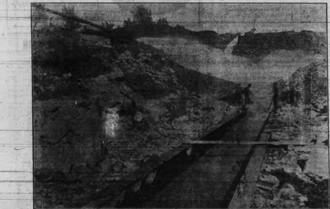
HYDRAULICING IN CARIBOO, SHOWING FLUME.
