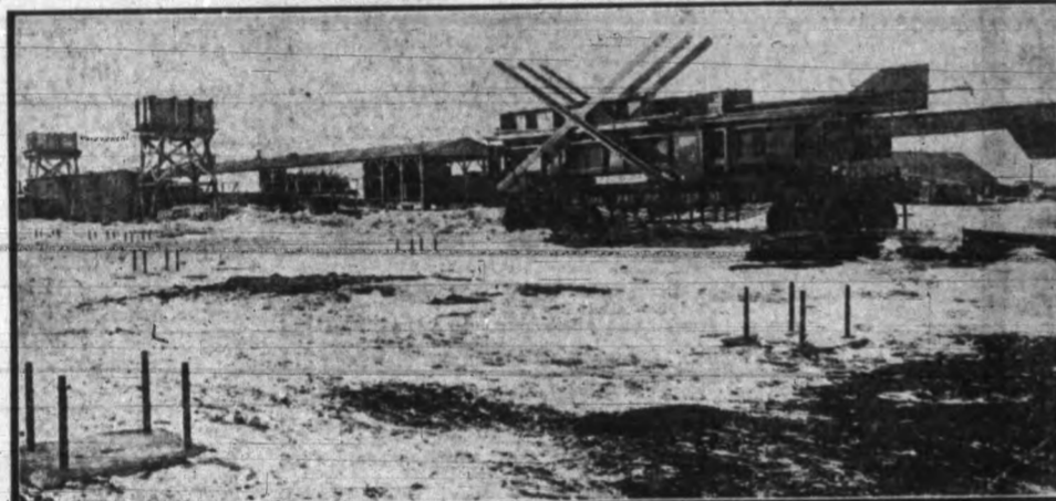
North of Locomotive Shops—Concrete Foundation for Columns for the Frog and Track Shop—Car of Steel Ready to Unload.
