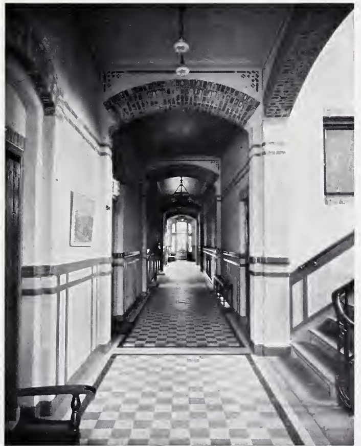
GANG 1STE VERDIEPING.
