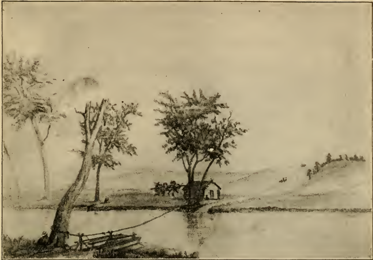
NEBRASKA FERRY ACROSS ELKHORN RIVER, 1854
