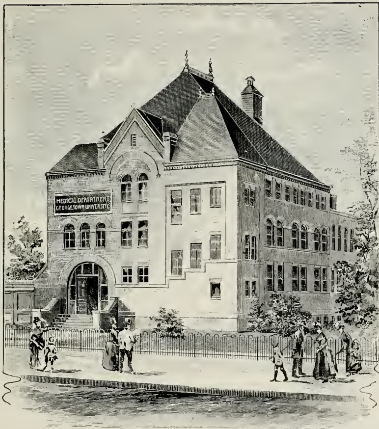
NEW BUILDING OF THE MEDICAL DEPARTMENT, H STREET, BETWEEN NINTH AND TENTH, N. W.
