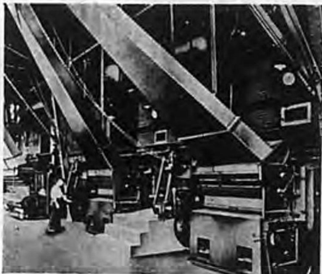
Patent Water Tube Boiler with Patent K.S.K. Stoker
