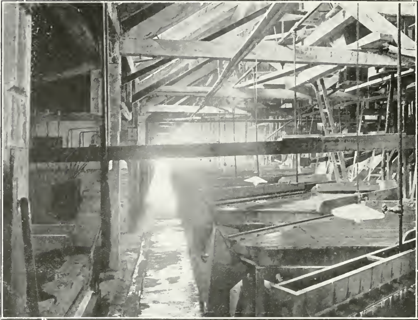
Sand Table Floor, Coniagas Concentrator.
