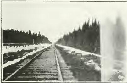
Looking east on the Transcontinental Railway, towards the Abitibi River, sixteen-mile tangent.
