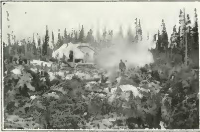
Burning off the right of way on the trunk road west of Cochrane.
