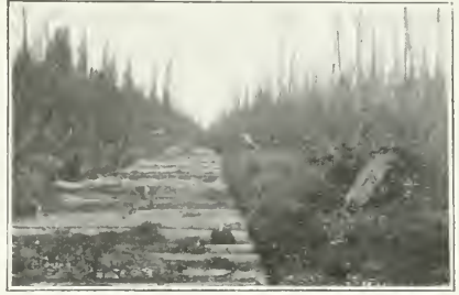
An unfinished corduroy road through semi-muskeg land.
