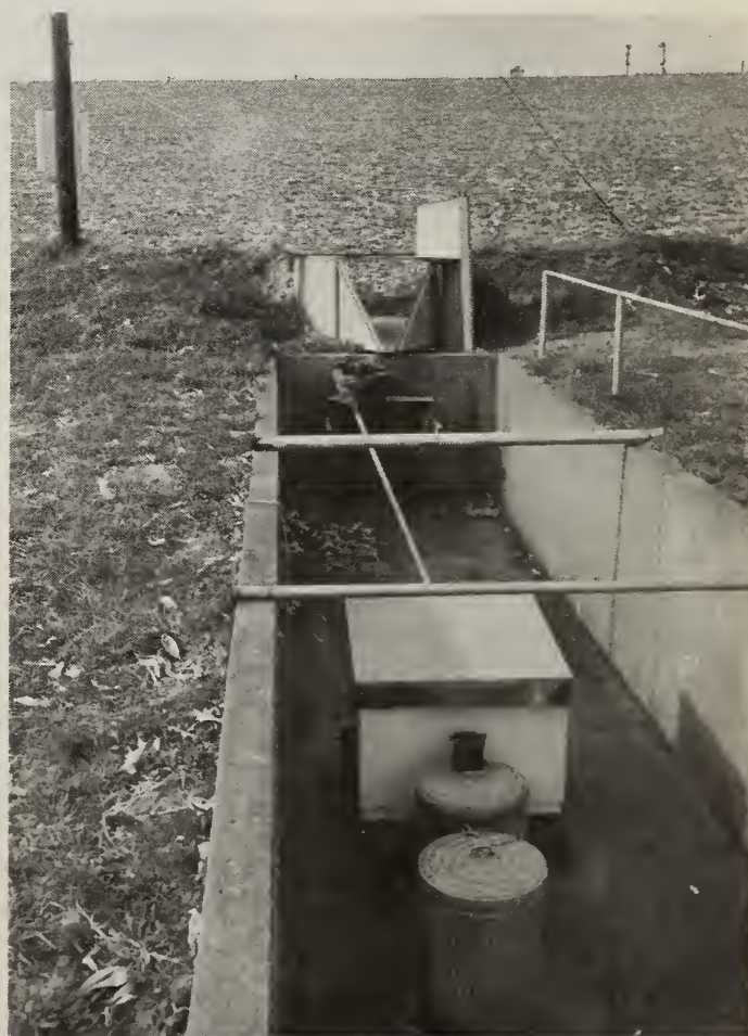
FIG. A-4.—Runoff gage and automatic flow sampler.
