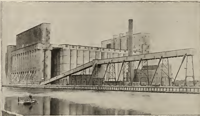
Chicago & North Western Railway Elevator South Chicago, Illinois Capacity 10,000,000 Bushels Completed 1920
