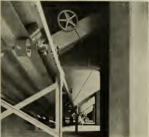
BIN BOTTOMS WITH CONVEYOR
