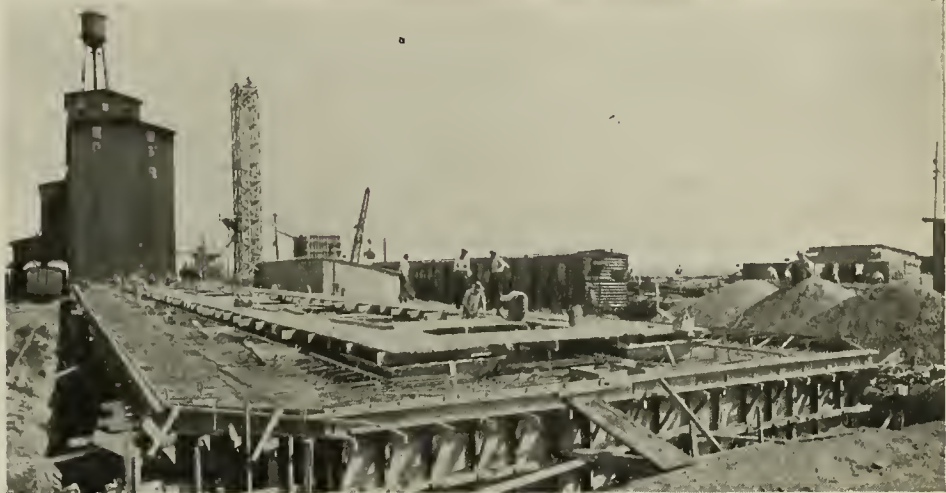
THE "MO-PAC" ELEVATOR'S 1,000,000-BUSHEL ADDITION
