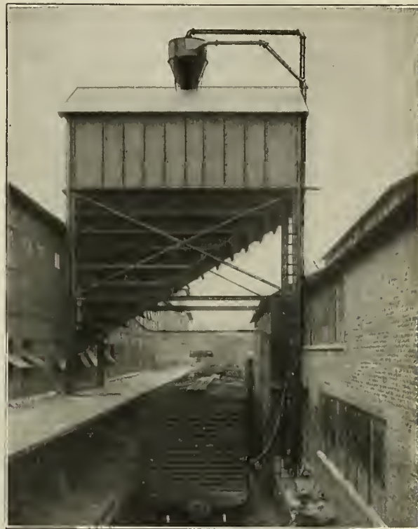
RECEIVER WHERE GRAIN IS SEPARATED FROM AIR
