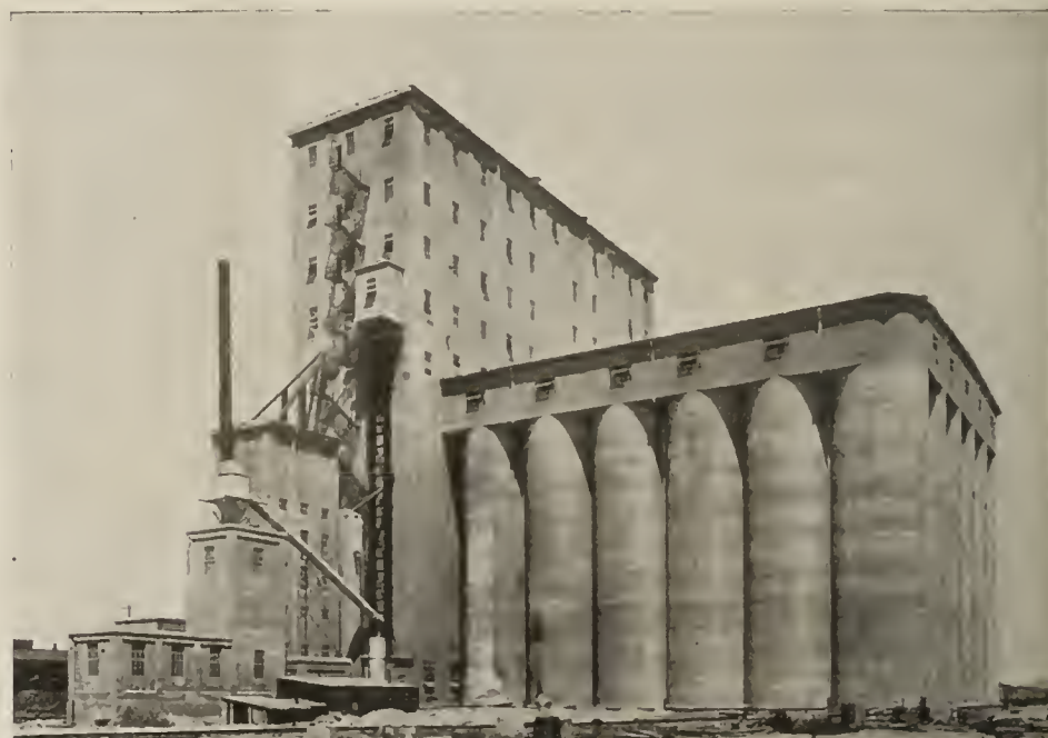
1,500,000-BUSHEL UPDIKE PLANT, COUNCIL BLUFFS
