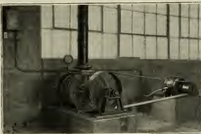
EXHAUST ARRANGEMENT FOR GRAIN UNLOADER
