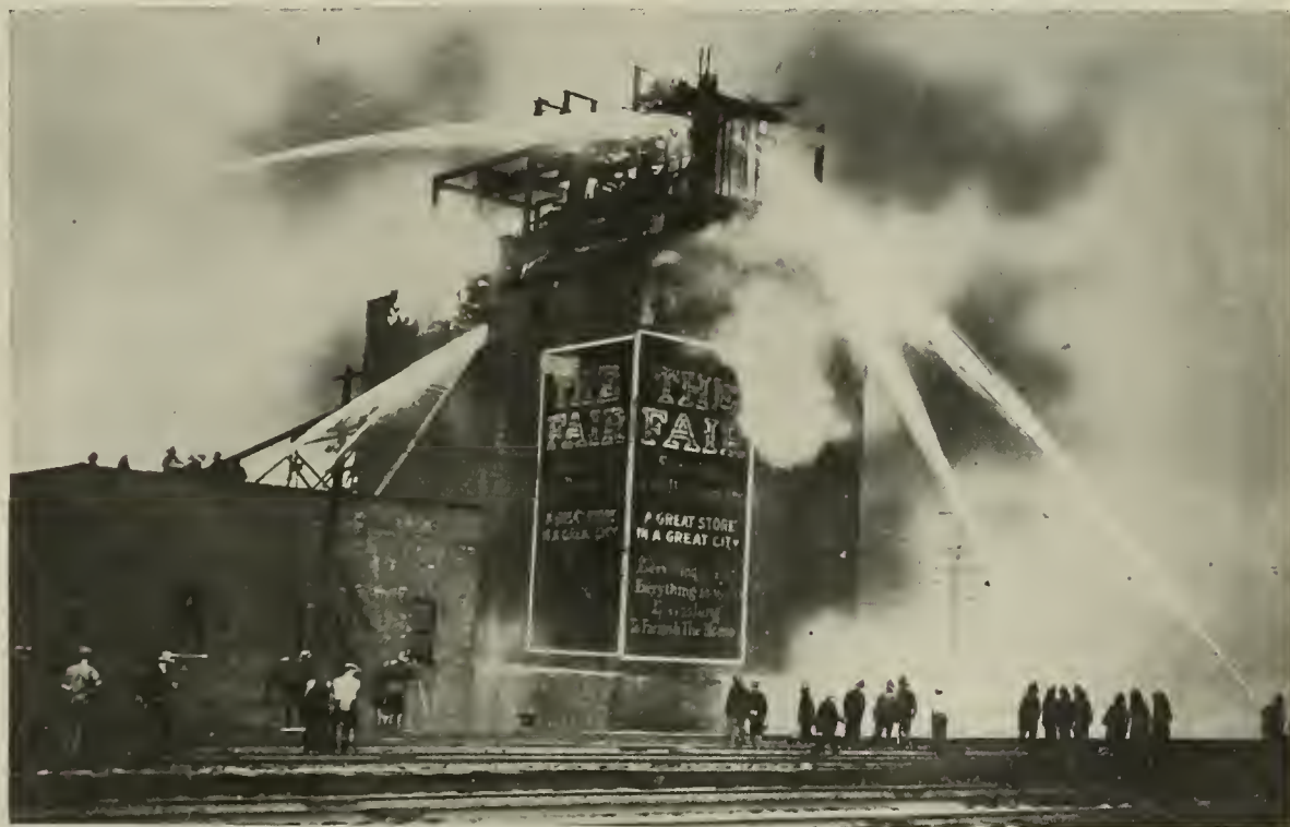
FIRE WHICH DAMAGED ELEVATOR OF THE WILLIAMS GRAIN COMPANY, CHICAGO
