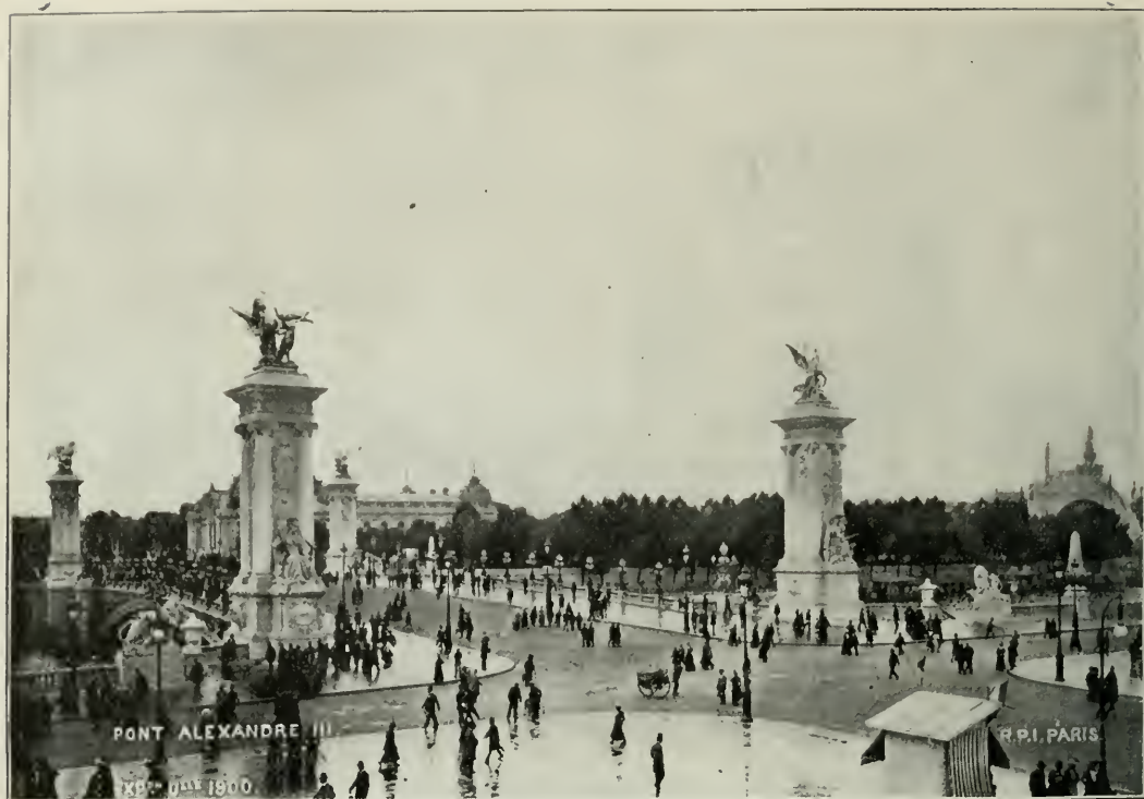
FIG. 2011. ALEXANDER III BRIDGE, PARIS.
