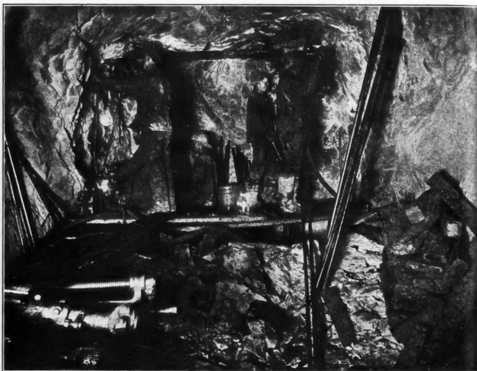
FIG. 1.—AT THE BREAST IN NEWHOUSE TUNNEL.
