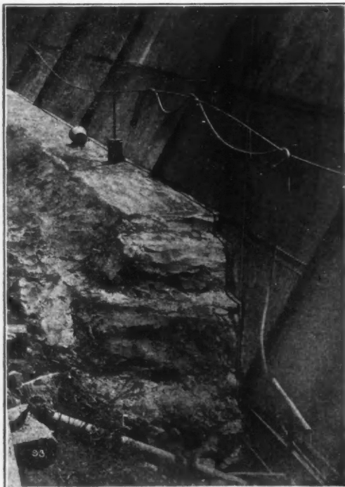
STEEL FACE OF DAM, SHOWING CONCRETE CONNECTION WITH BED-ROCK.
