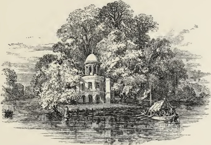
ISLAND, FAWLEY COURT.
