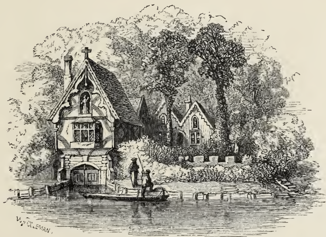
THE BOAT-HOUSE AT PARK PLACE.
