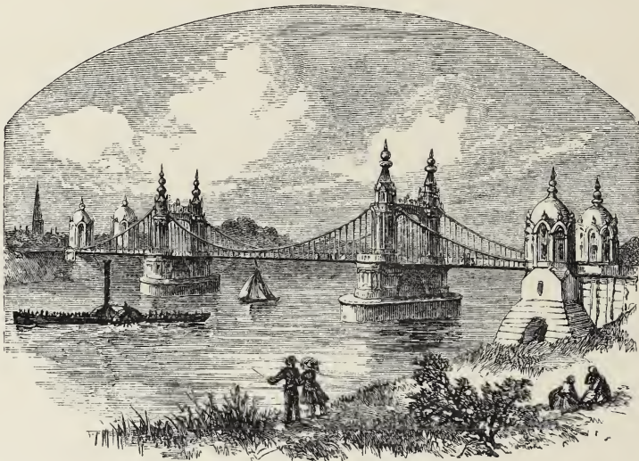
THE NEW BRIDGE AT CHELSEA.
